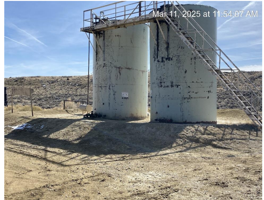
No sign at tank battery
