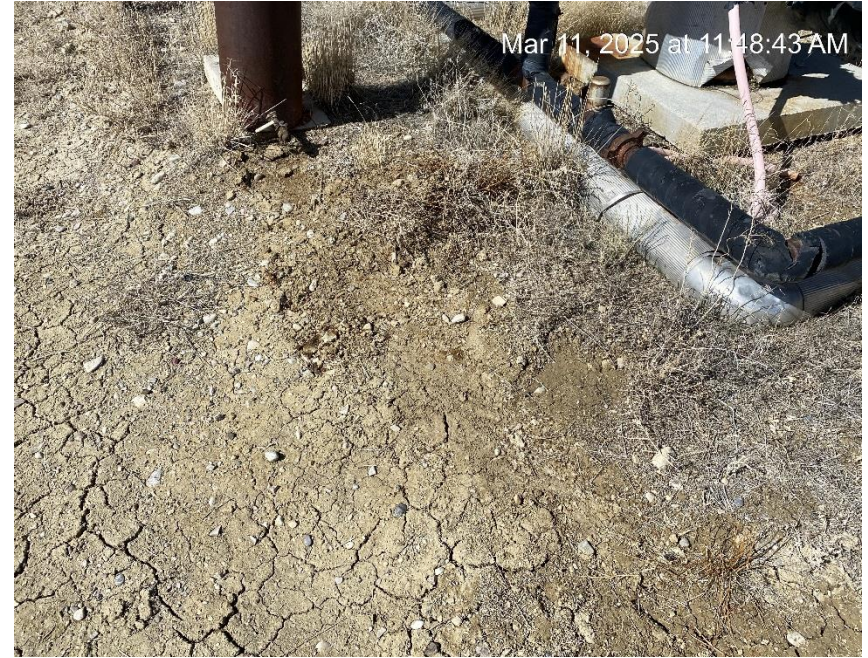
Oily waste and contaminated soil.
