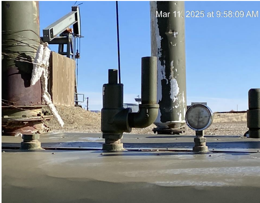
Unprotected relief riser
