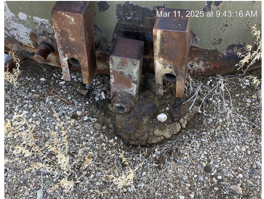
Oily waste. Staining
