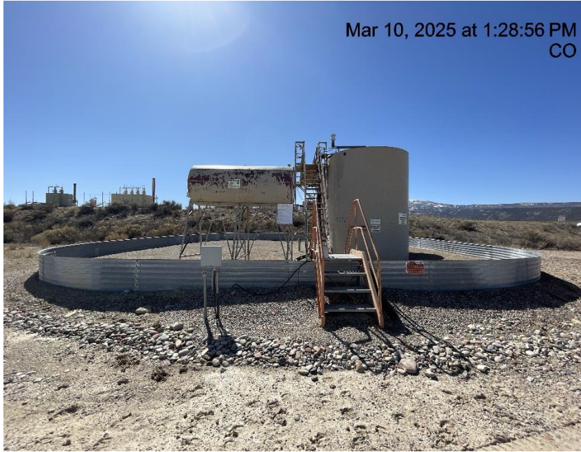
Photo # 1962 Battery lacks required signage
