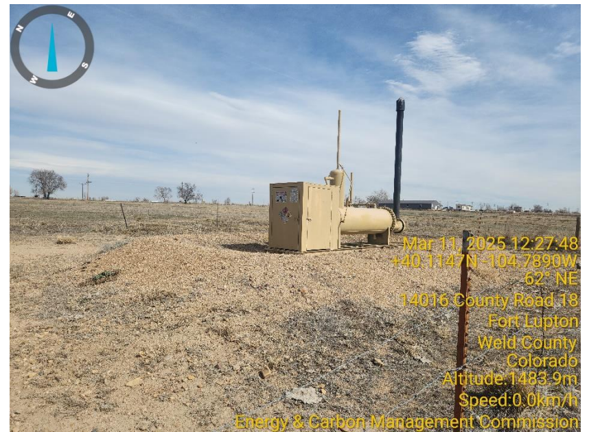
Photo 10 Horizontal Heated separator.
