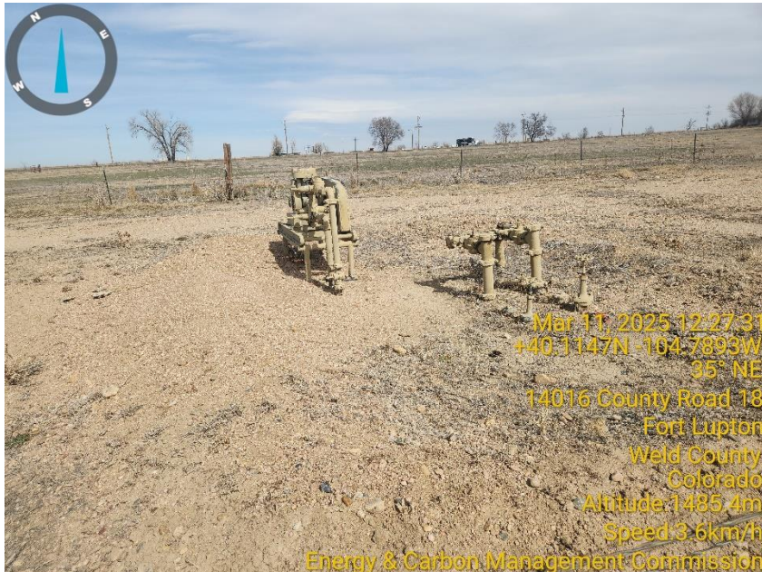
Photo 9 flow line manifold.
