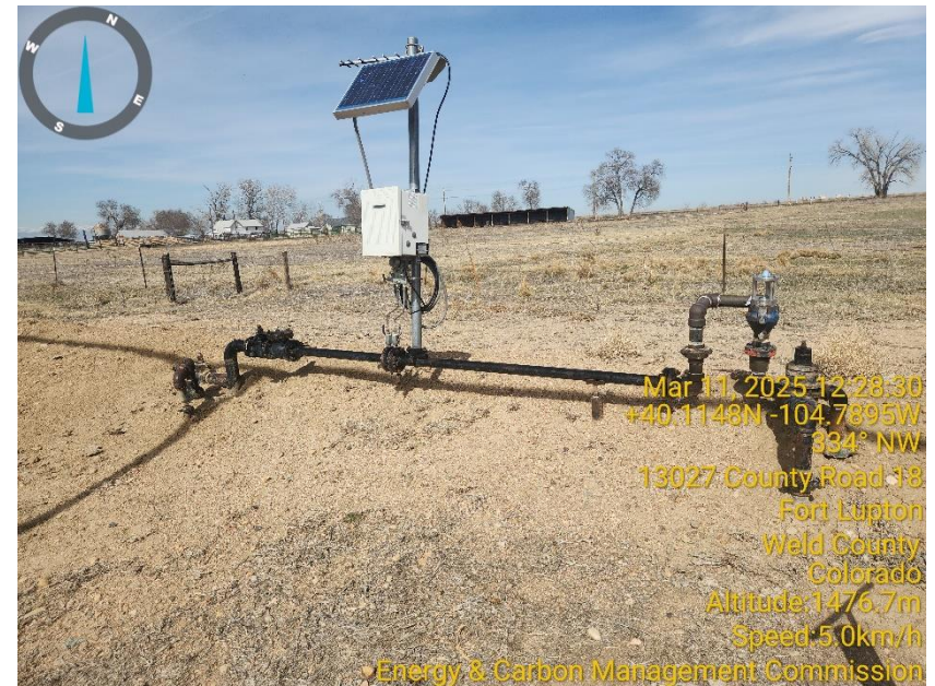
Photo 8 Gas Meter Run.
