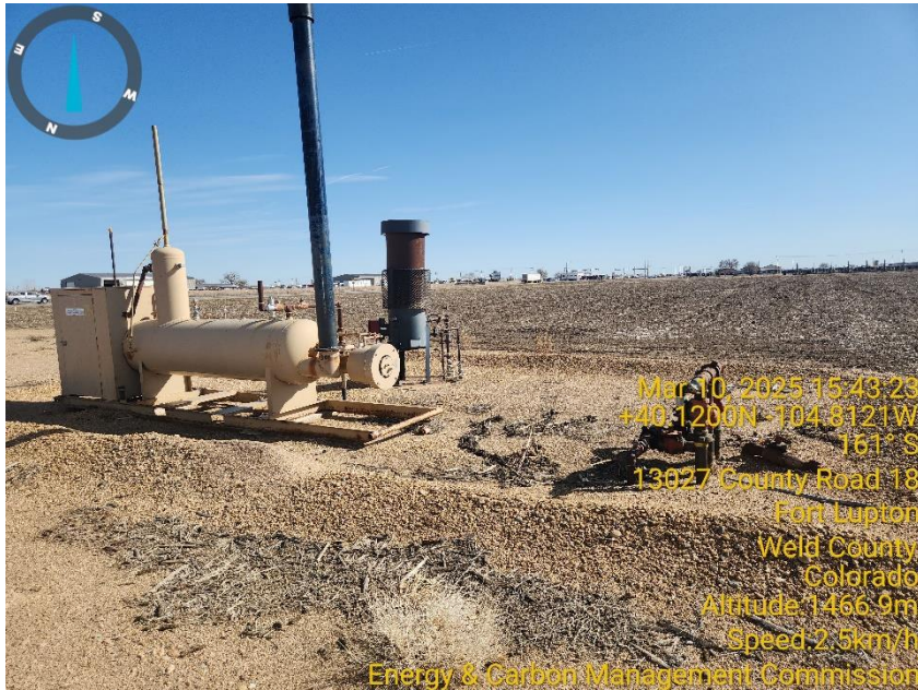
Photo 5 Flow line manifold, ECD & Horizontal Heated Separator.
