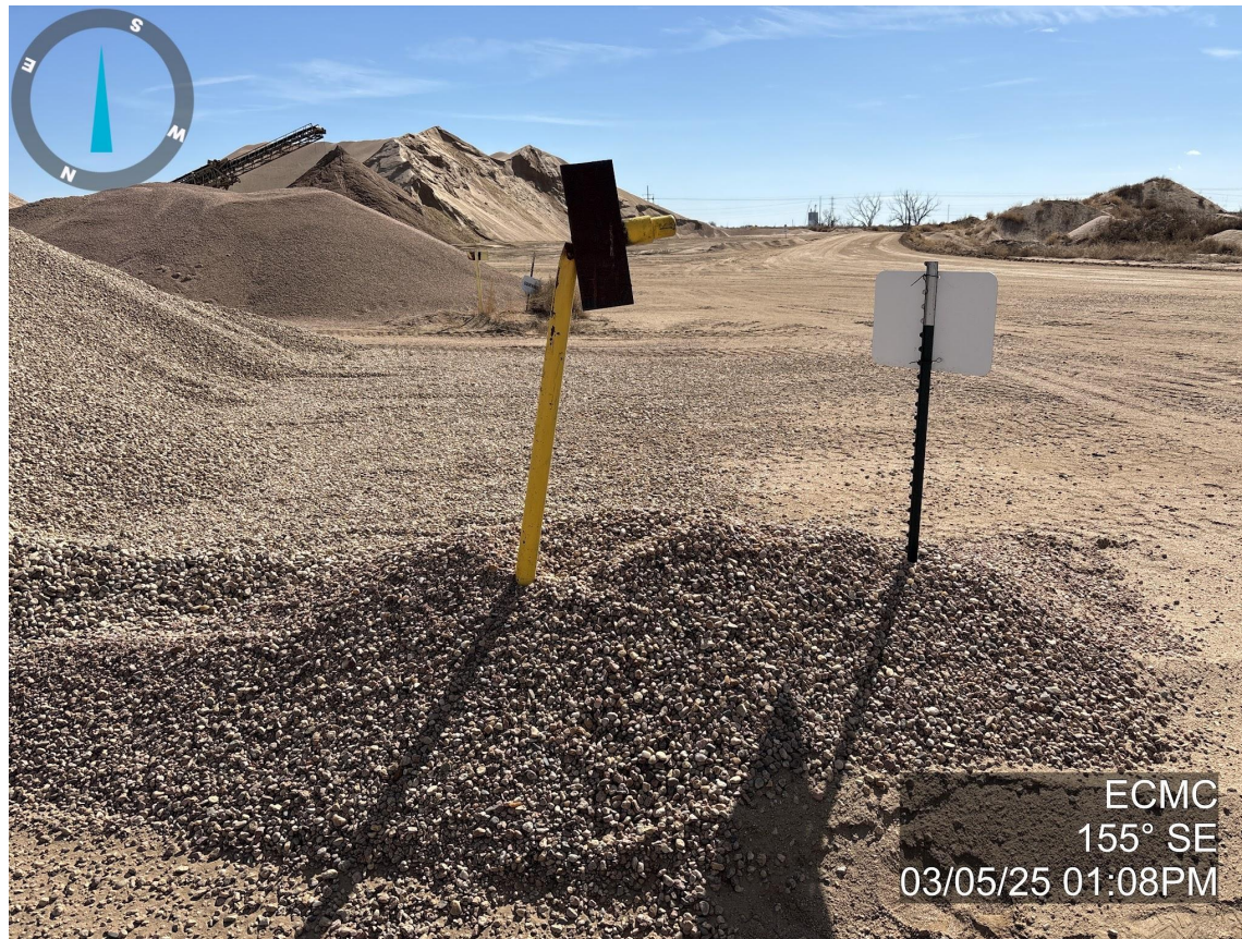
Photo 3. Photo taken from the THOMPSON #23-6 well location, facing Southeast. Photo illustrates that all equipment and stormwater BMPs have been removed and there is no weed growth on the well location. The well location is in a land-use change to an active Gravel Mine, Mine ID M2018027.
