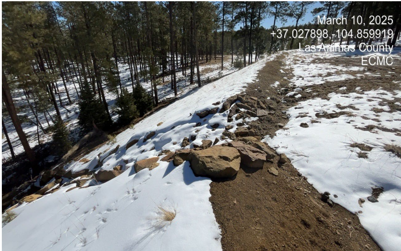
Photo 2. Facing toward the fill slope with a rip/rap stormwater outlet..
