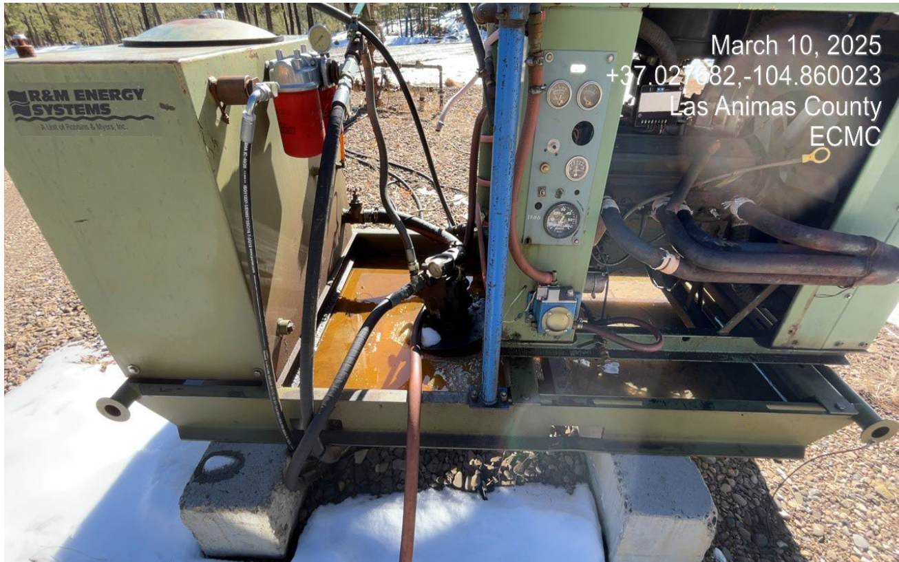
Photo 3. There is oily fluids in the engine skid that needs to be cleaned up.
