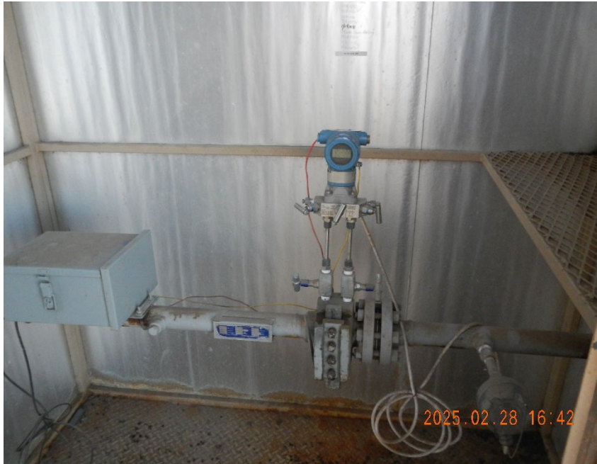
5. Gas meter inside meter shed.
