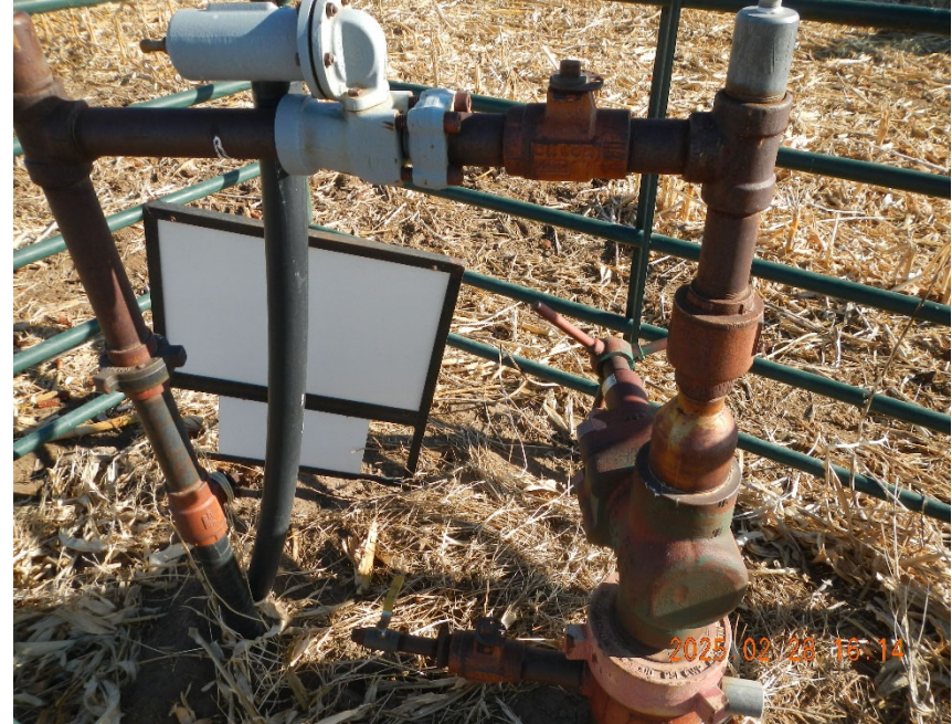
2. View of wellhead. Open ended black poly line noted.
