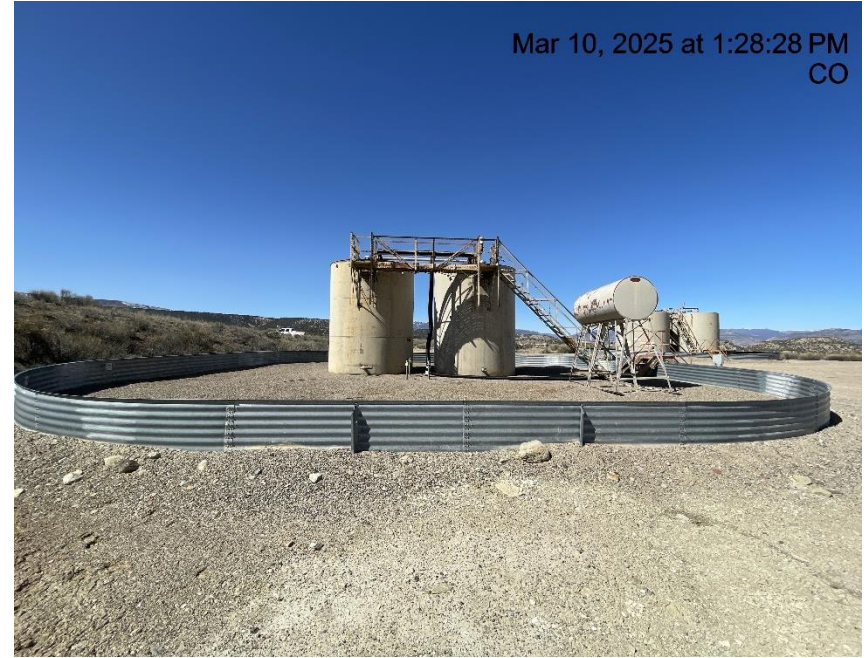
Photo # 1963 Battery lacks required signage
