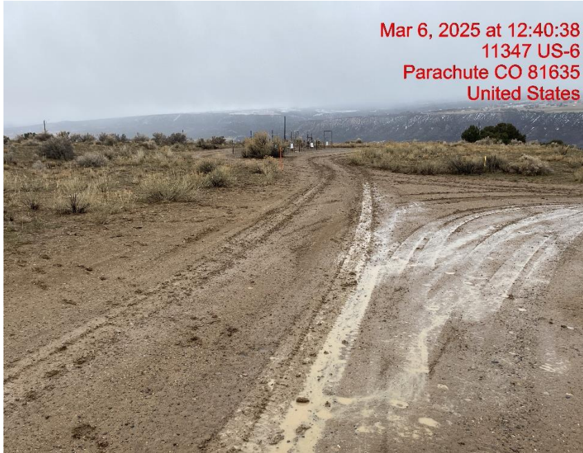
Lack of Stabilization – Photo #07118
