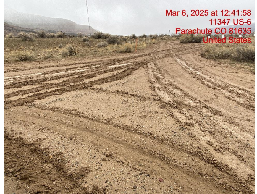
Lack of Stabilization – Photo #07120
