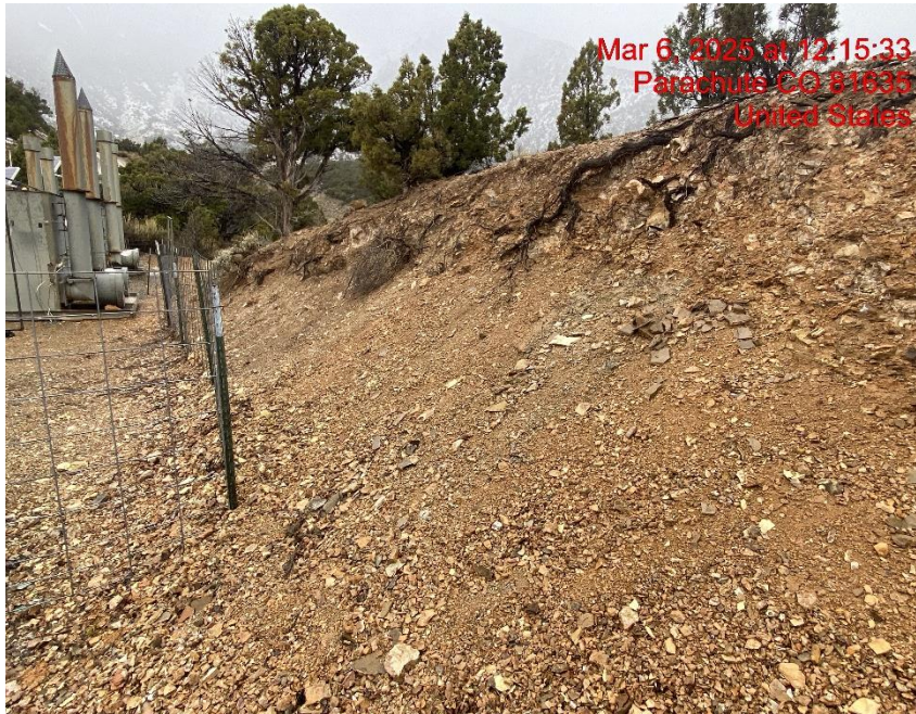
Insufficient Erosion Control – Photo #07094
