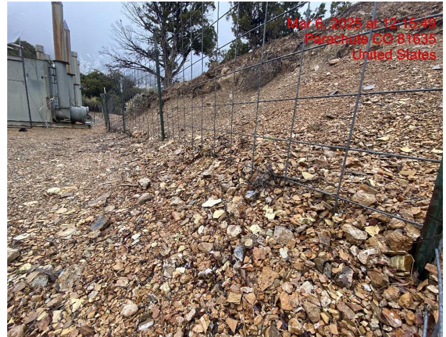
Insufficient Erosion Control – Photo #07095
