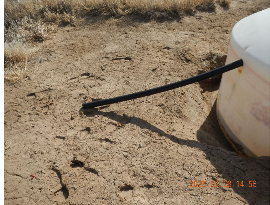
8. Closer view of overflow line that crosses top of tank berm.
