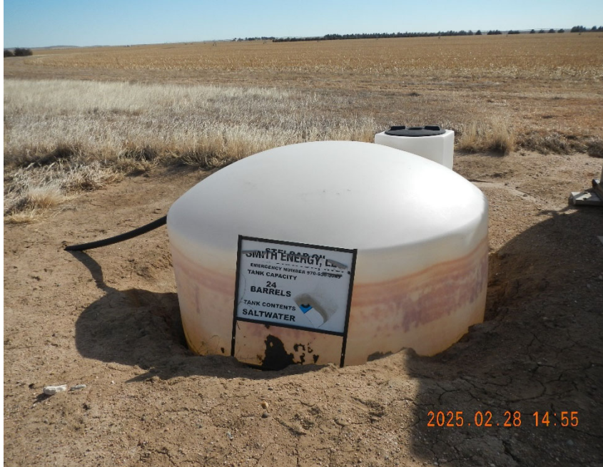
7. Overview of produced water tank. Note overflow line left side of tank.
