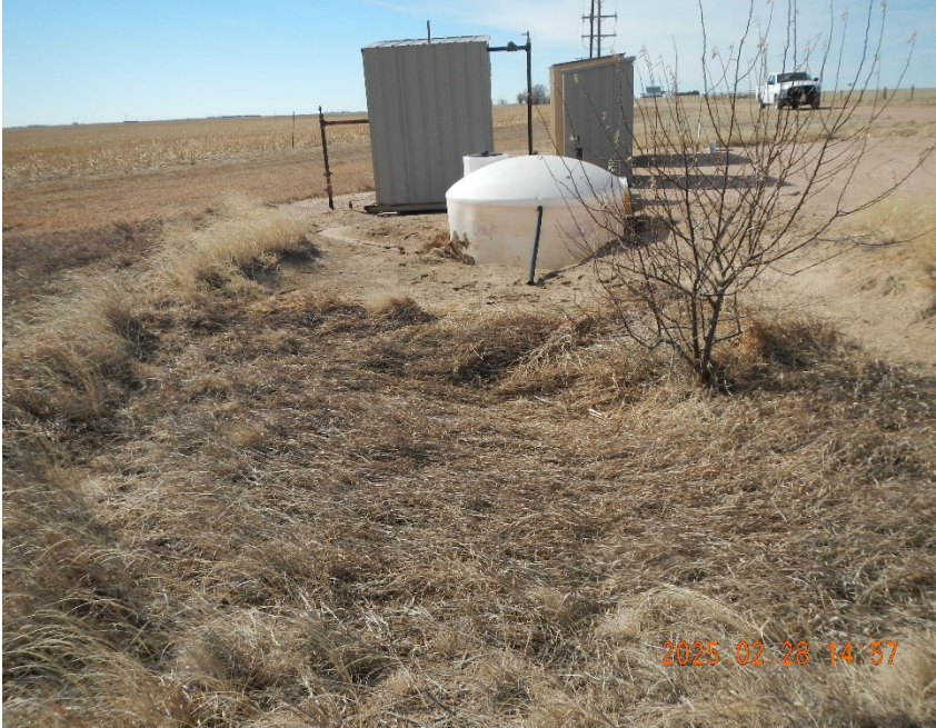
9. View of approximately 15' X 15' overflow pit located at gathering/production facility.
