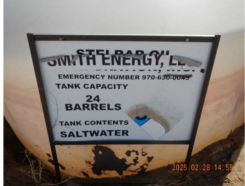
6. View of Content/Quantity/Hazard sign at produced water tank. Part of sign is unreadable and operator sticker is peeling.
