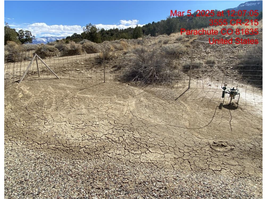
Insufficient Erosion Control – Photo #07069
