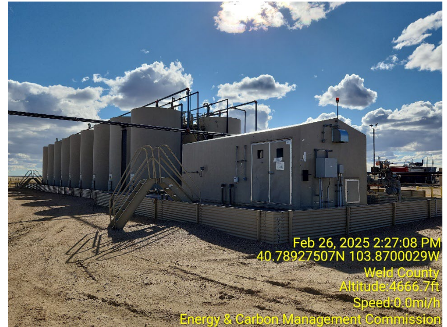
Photo 4 – Tank Battery and LACT
