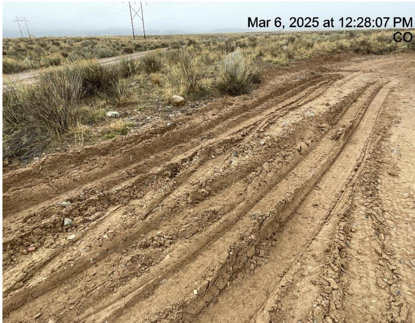
Photo # 1315 Lack of stabilization/compaction on location /insufficient BMP's
