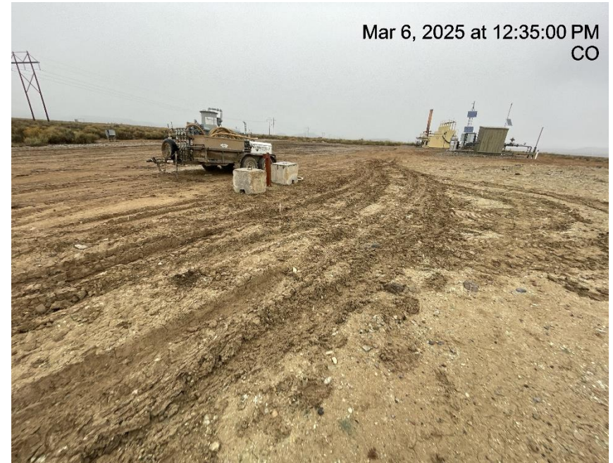
Photo # 1318 Lack of stabilization/compaction on location /insufficient BMP's
