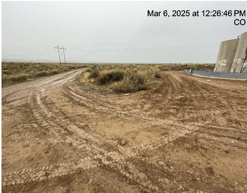
Photo # 1313 Lack of stabilization/compaction on location & tracking onto lease road/insufficient BMP's
