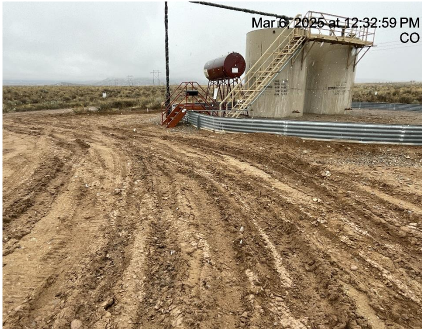
Photo # 1317 Lack of stabilization/compaction on location & tracking onto lease road/insufficient BMP's
