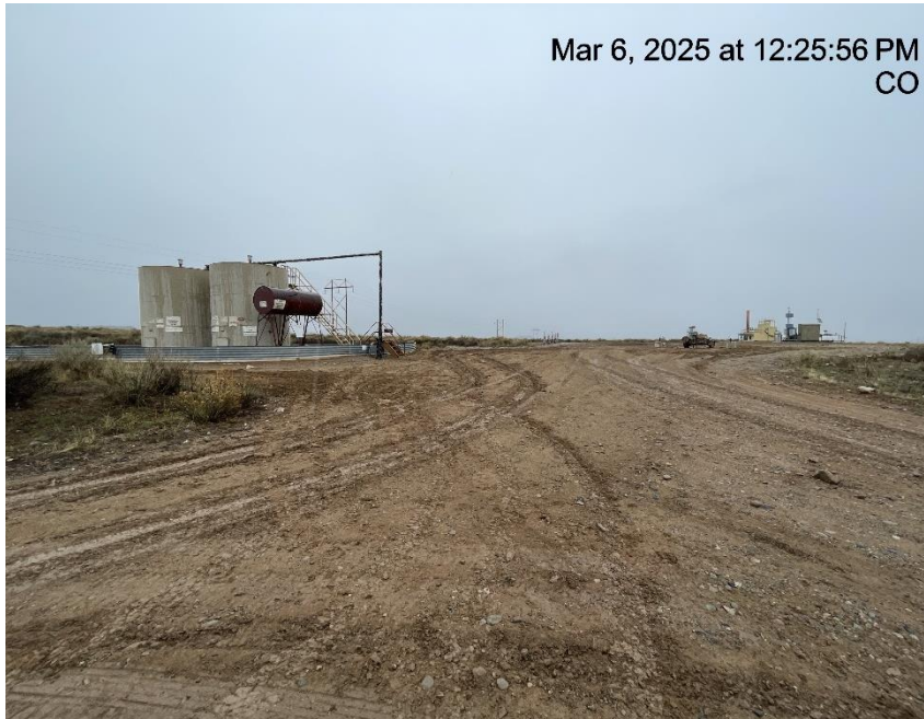
Photo # 1311 Lack of stabilization/compaction on location & tracking onto lease road/insufficient BMP's
