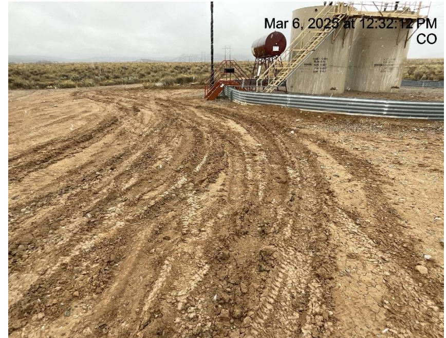
Photo # 1316 Lack of stabilization/compaction on location & tracking onto lease road/insufficient BMP's
