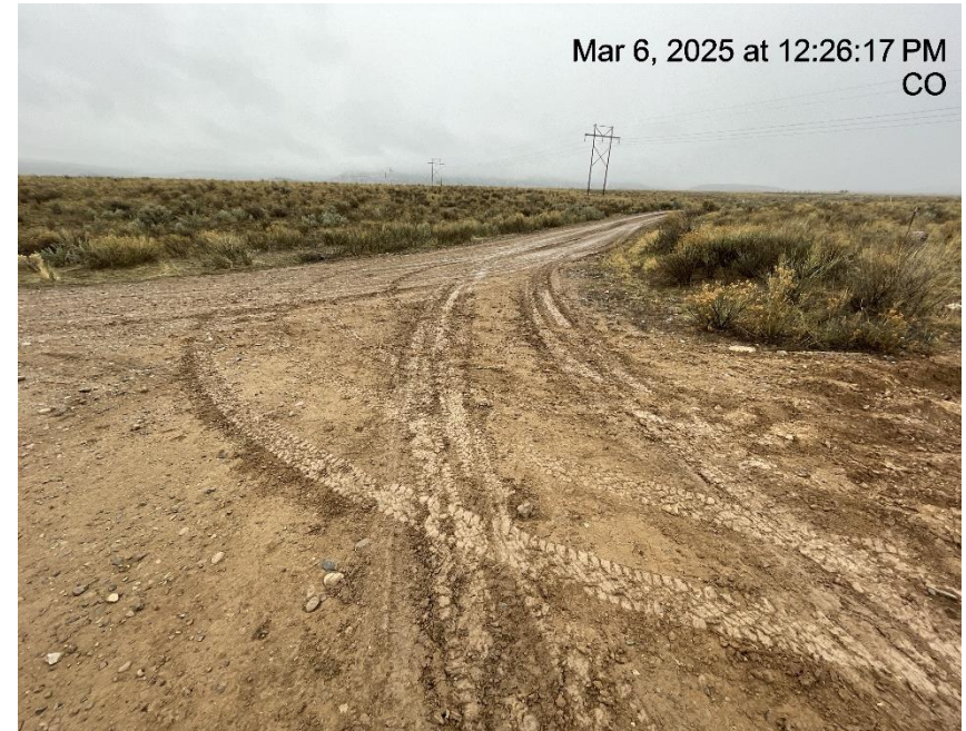
Photo # 1312 Lack of stabilization/compaction on location & tracking onto lease road/insufficient BMP's
