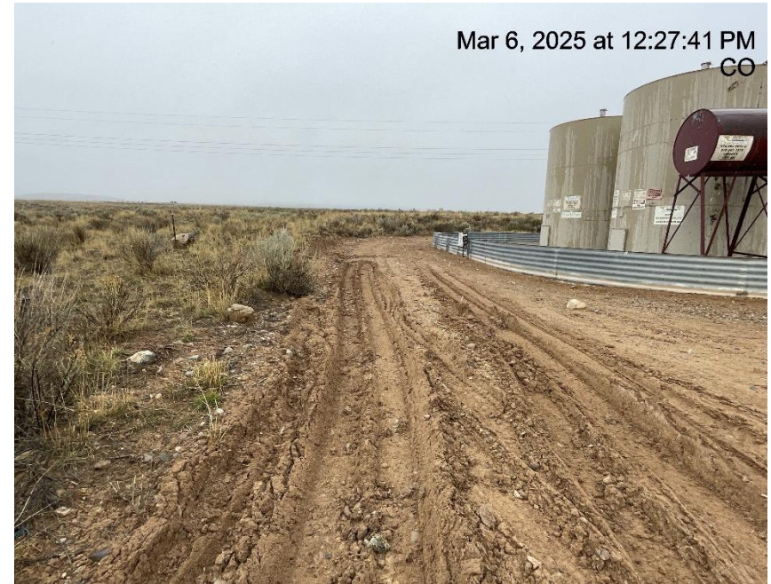
Photo # 1314 Lack of stabilization/compaction on location /insufficient BMP's
