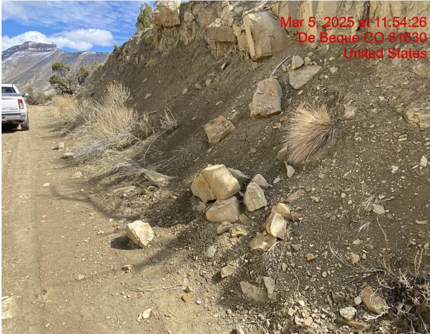
Insufficient Erosion Control/Degradation – Photo #07060
