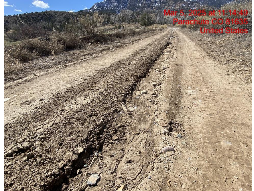
Rill Erosion Cutting Through Lease Road – Photo #07043
