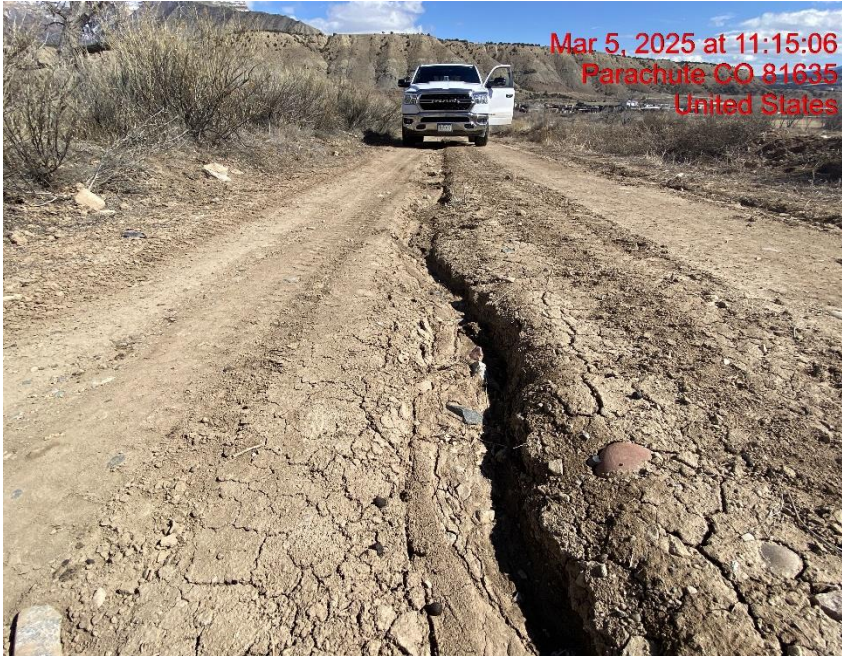
Rill Erosion Cutting Through Lease Road – Photo #07044
