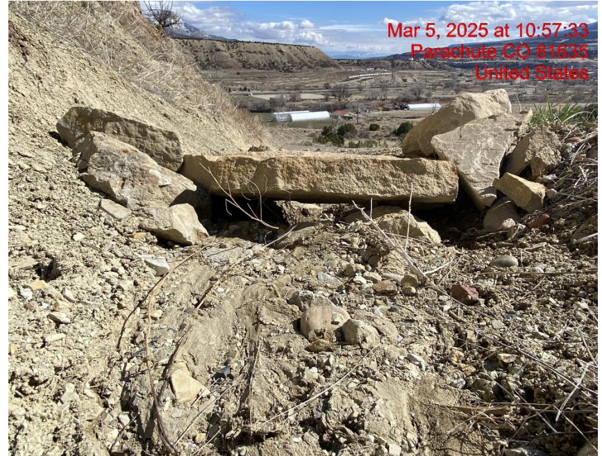
Check Dam BMP Needs Maintained – Photo #07025
