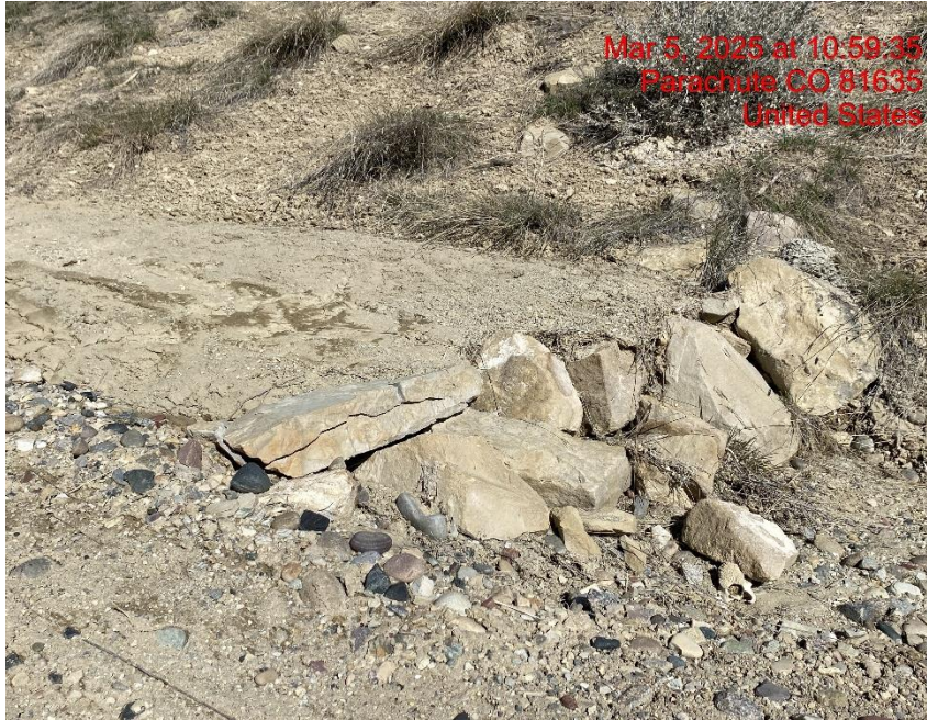
Check Dam BMP Needs Maintained – Photo #07028
