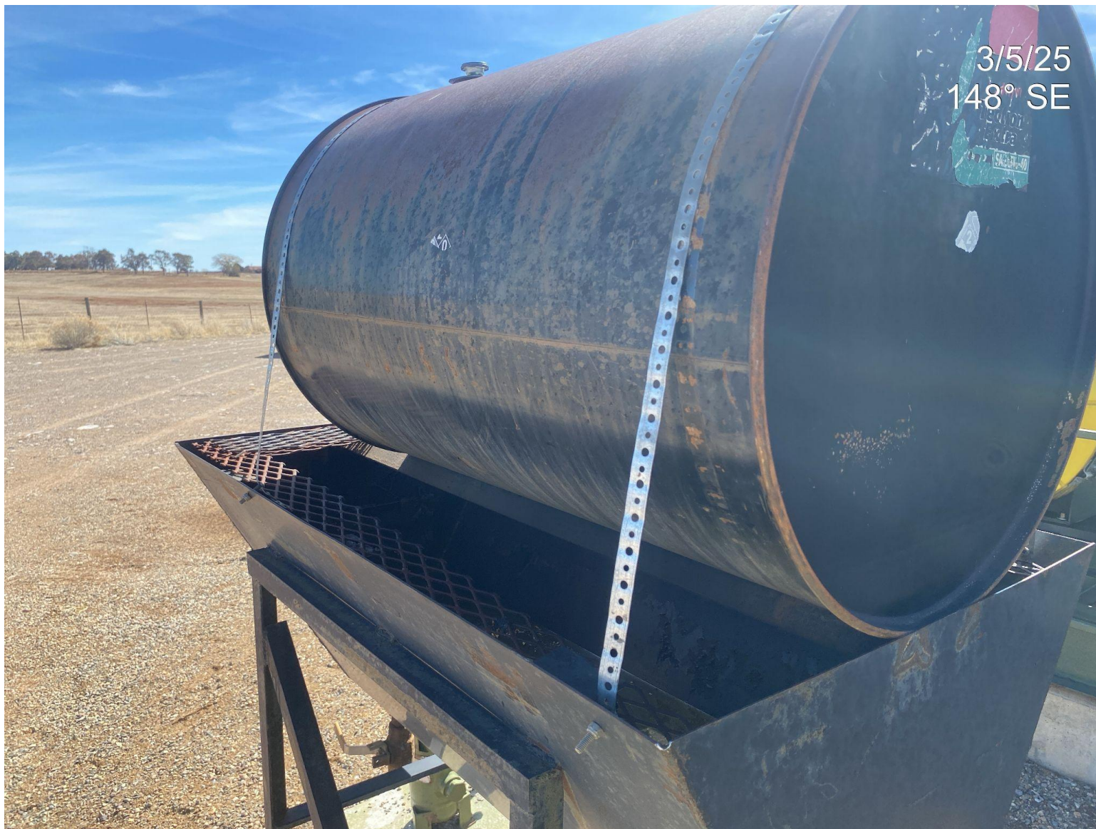
Photo 3. Wildlife covering/BMP at lube tank secondary containment has gaps and is not functioning.
