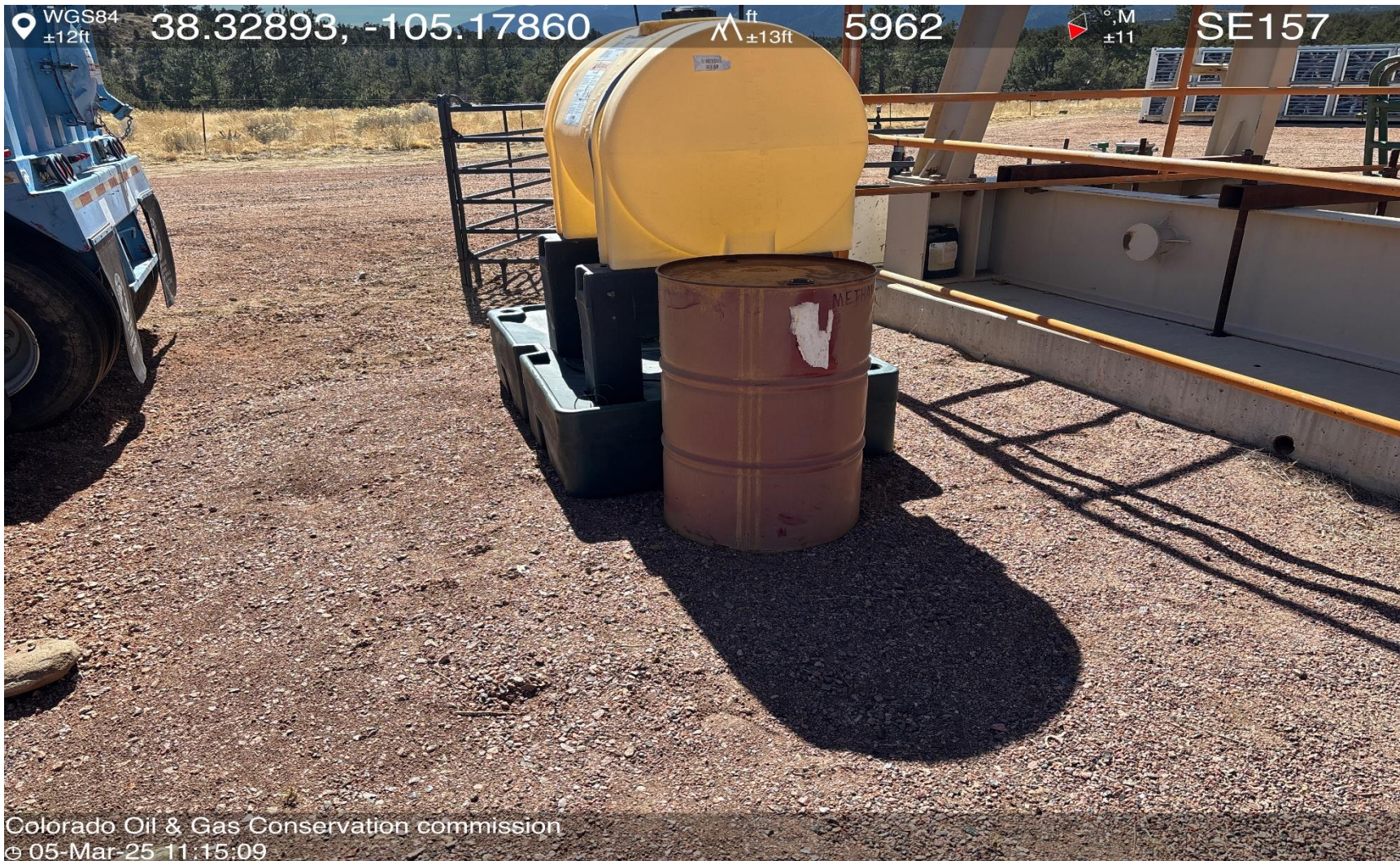
PHOTO 7: 55 GAL METHANOL TANK NOT IN SECONDARY CONTAINMENT. Non E&P Waste not properly stored, handled, transported, treated, or disposed per Rule 906. Contact COGCC EPS staff. Require appropriate cleanup. CA DATE 3/10/2025.
