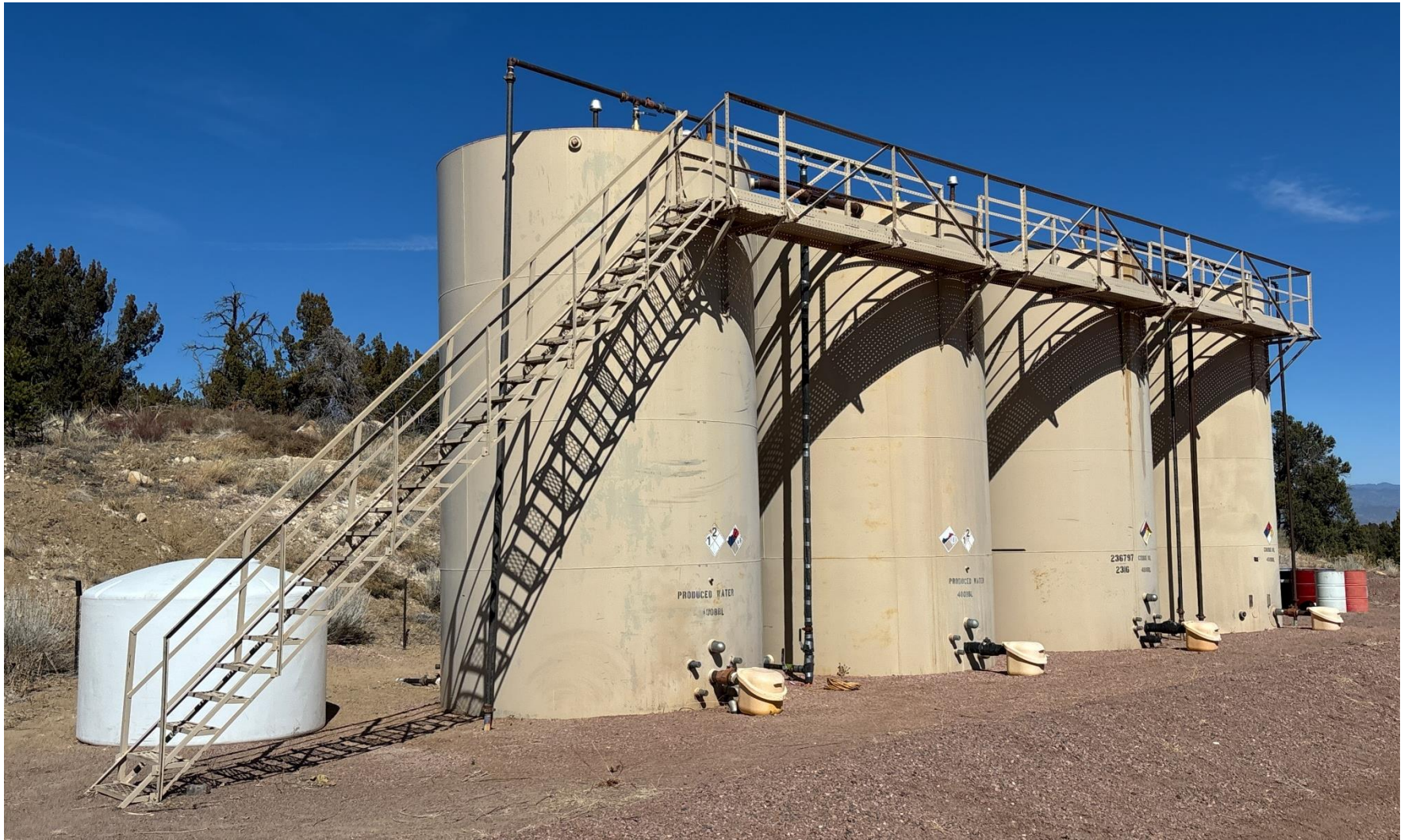
PHOTO 4: PERMAMENT TANK BATTERY.
