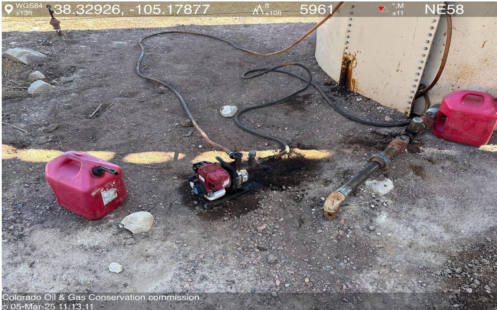
PHOTO 10: AREA OF IMPACTED SOIL FROM LEAKING PUMP ON NORTHERN MOST PERMENANT TANK BATTERY. Conduct maintenance on equipment, cleanup stained material and review self inspection processes. COMPLY WITH RULE 1002,(2).DCA DATE 3/10/2025.
