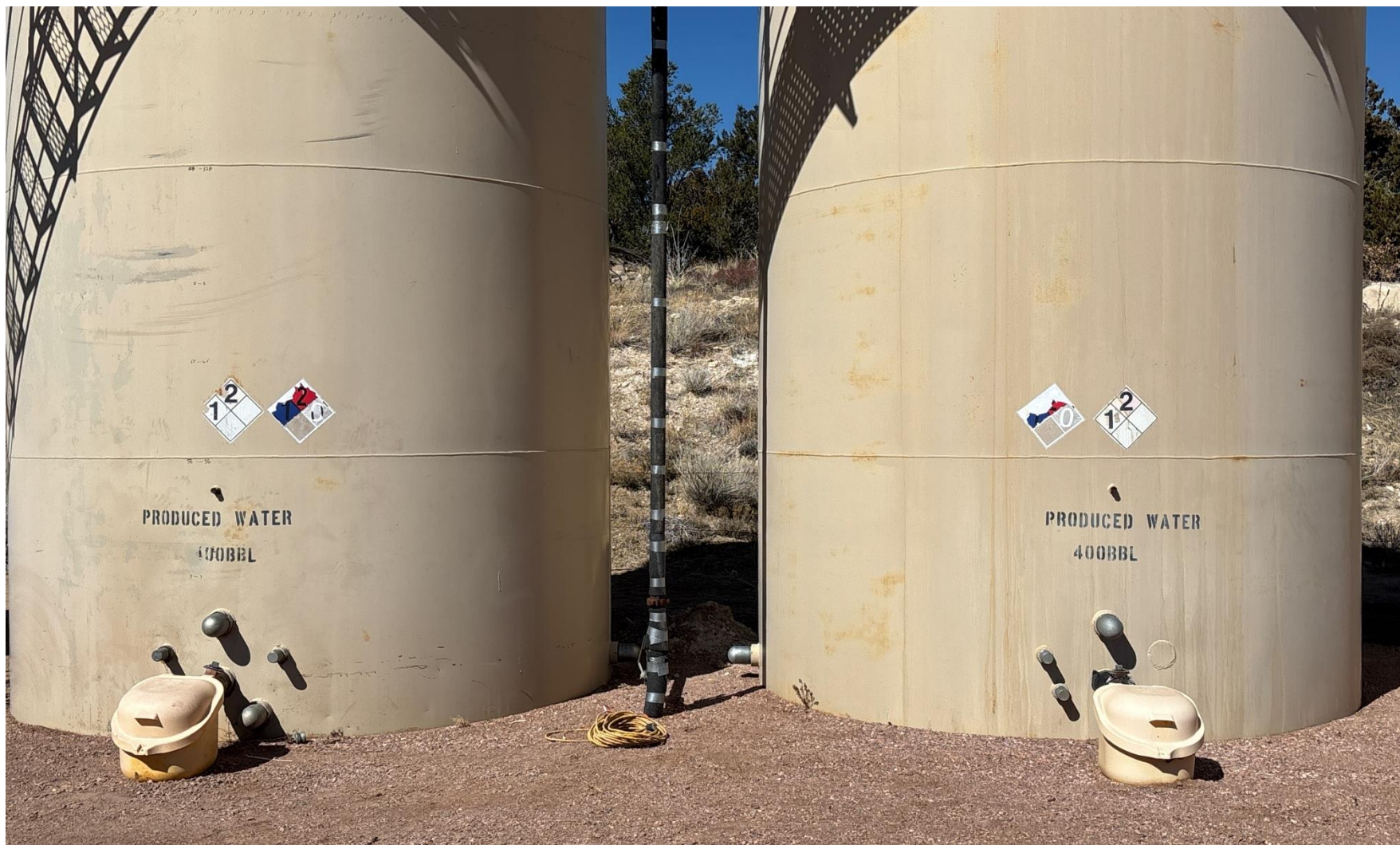
PHOTO 8: NFPA STICKERS ARE FADING AND PEELING. Install sign to comply with Rule 605.h. CA DATE 3/10/2025.
