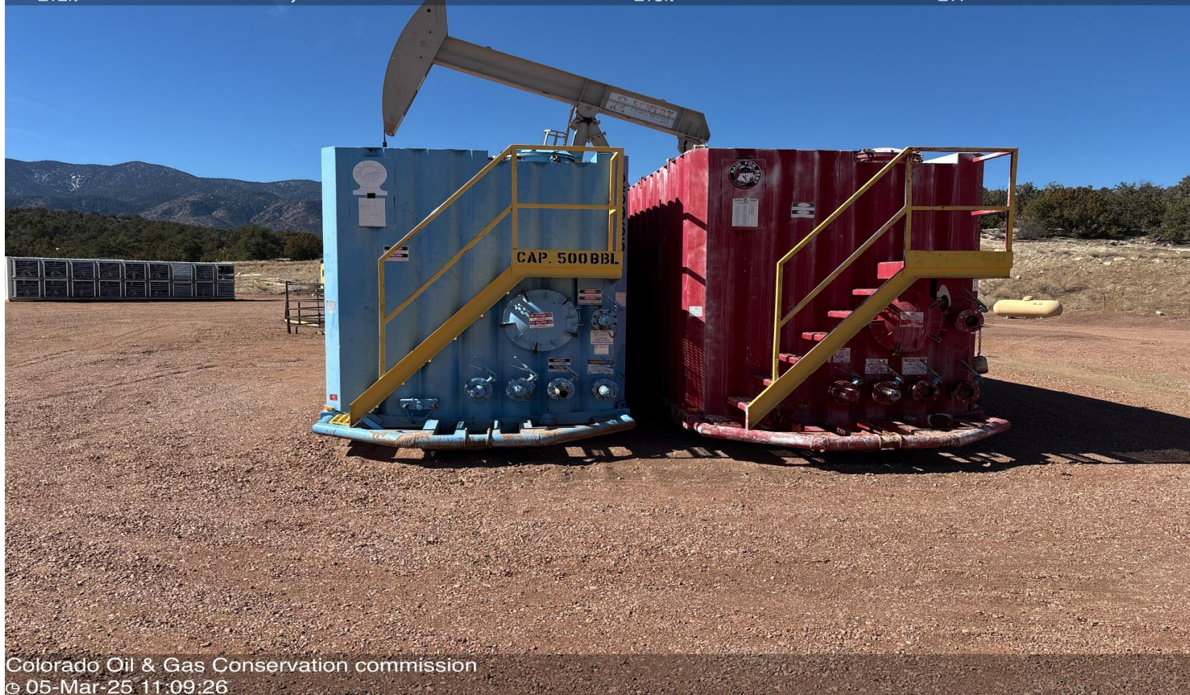
PHOTO 5: TEMPORARY TANK BATTERY HAS NO NFPA STICKERS, NEATHER TANK HAS CONTENTS POSTED AND ONE TANK DOES NOT HAVE CAPACITY POSTED. Install sign to comply with Rule 605.h. CA DATE 4/5/2025.
