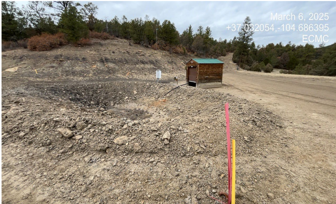
Photo 1. Facing southwest toward the PW pit which has been dug out to accommodate 2 ft. freeboard.
