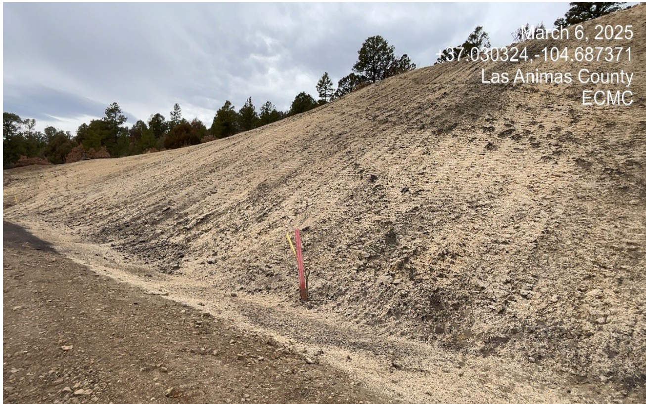
Photo 3. The cut slope has been reseeded and hydromulched.
