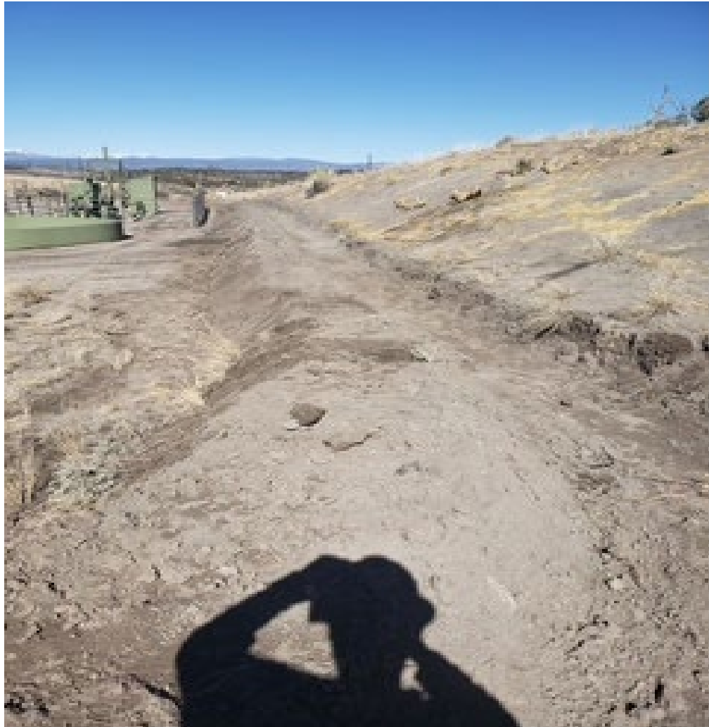
Runoff ditch cleaned out and tank label installed
