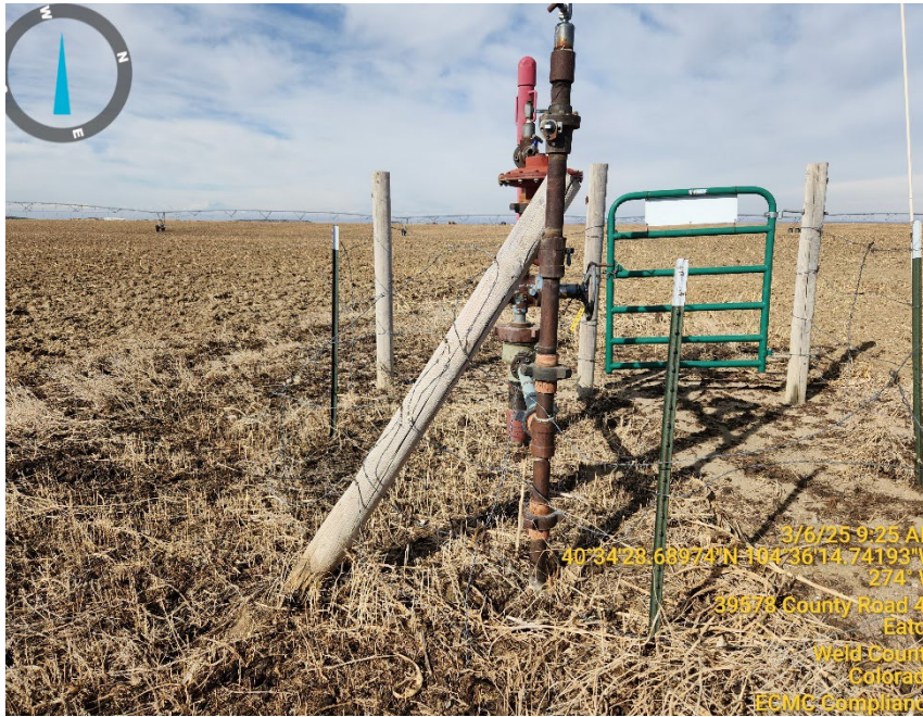
Photo 3: Fencing in disrepair
