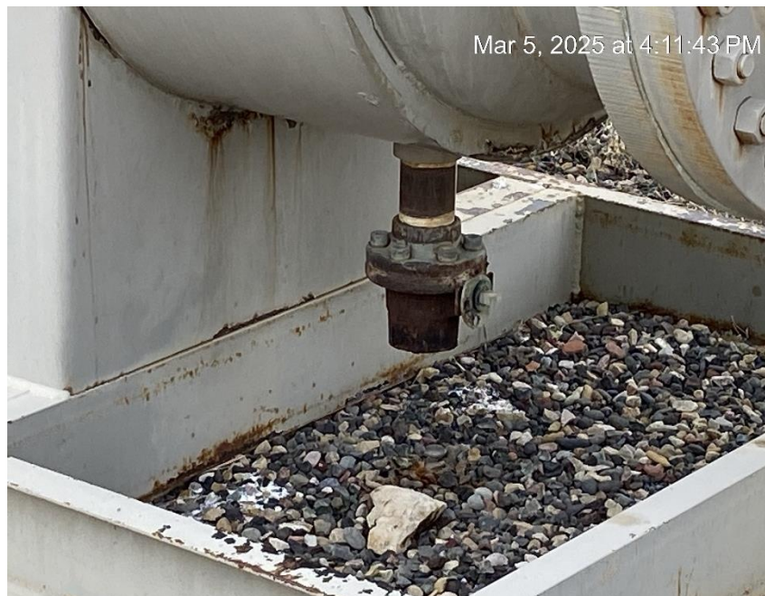
Drain valve plug missing
