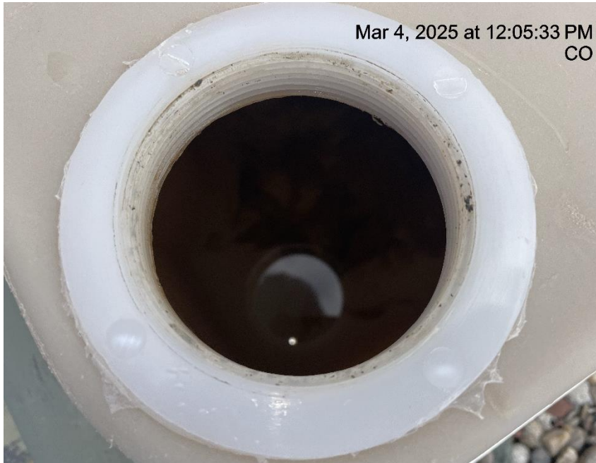
Photo # 552 Failure to maintain chemical BMP - Chemical tank containment approximately 2/3 to 3/4 full of fluid/BMP insufficient to contain possible spill
