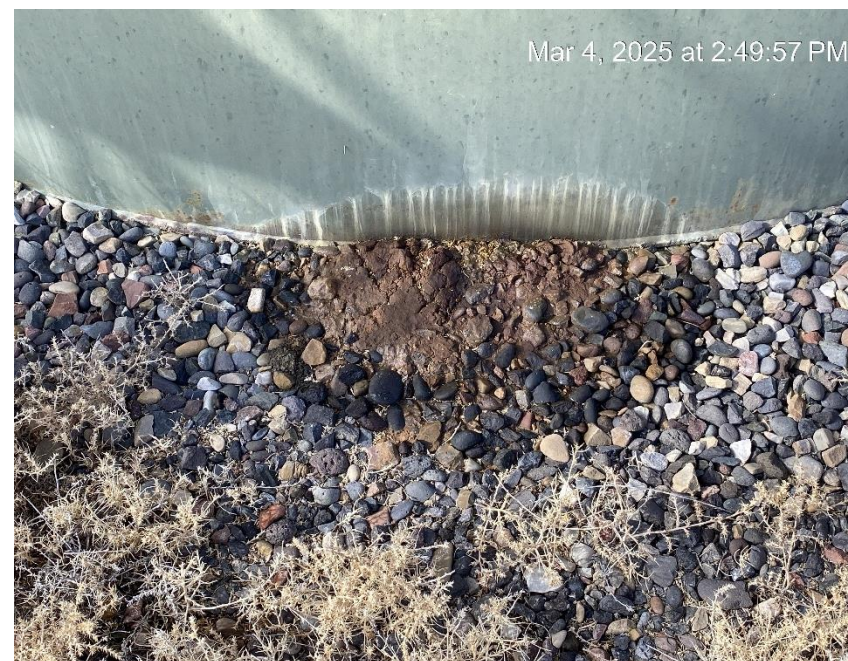
Tank leak
