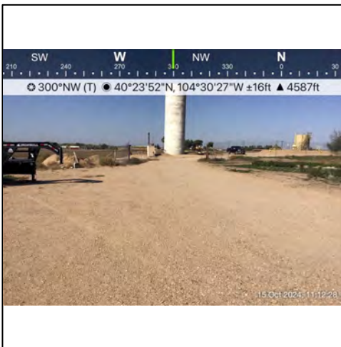
P7 - Looking west along the former access road, now being used as a farm access road.
