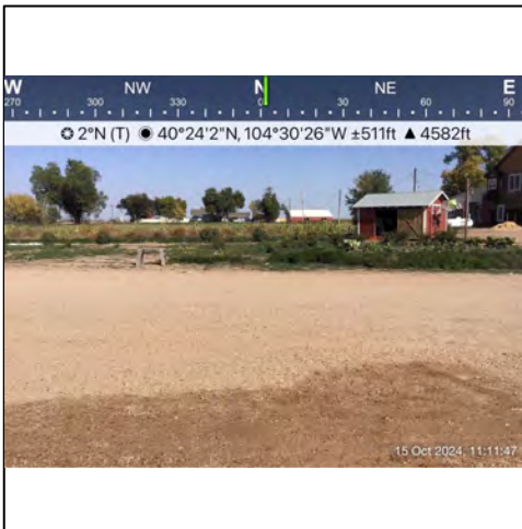
P1 - Looking north from the center of the Site, road base has been left in place per land owner request.
