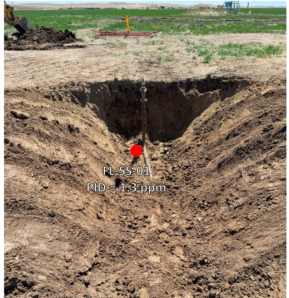
Looking east at flowline Pt A
