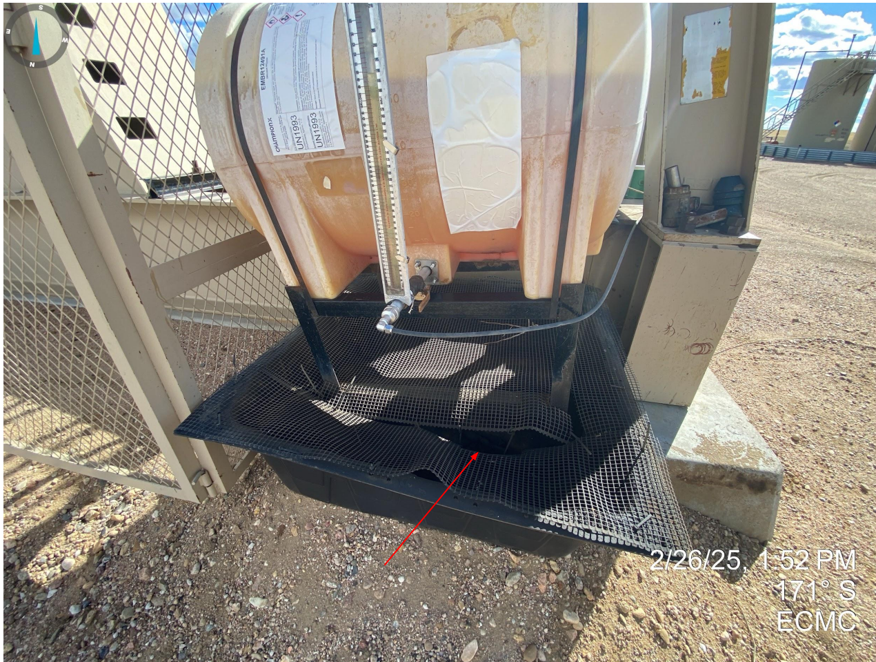
Photo 5. Wildlife netting inadequate at day tank.
