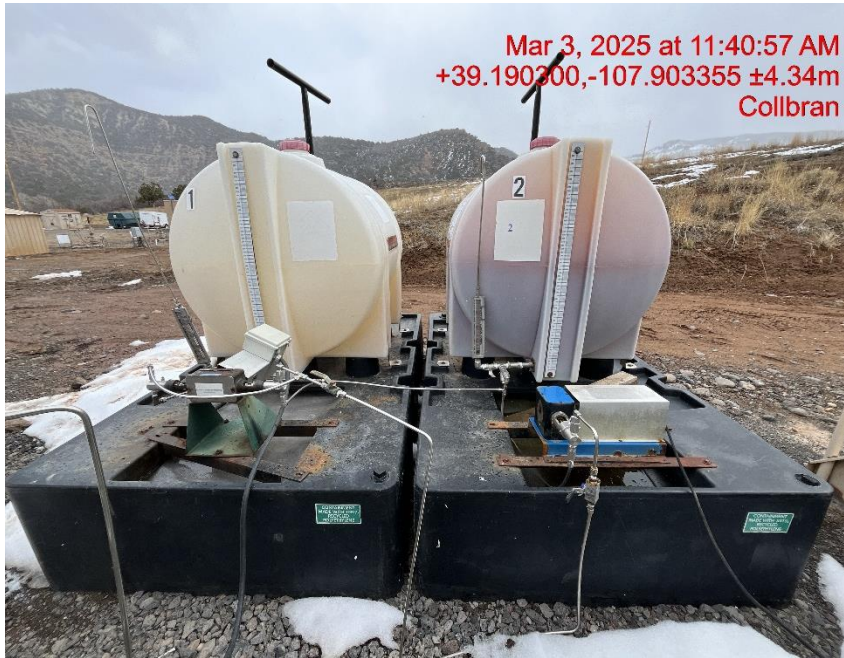
Photo # 6190 Failure to maintain chemical BMP's/chemical containments full of fluid & not sufficient to contain possible spill
