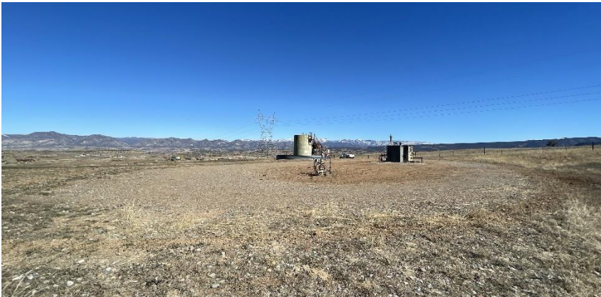
South West corner of location.
