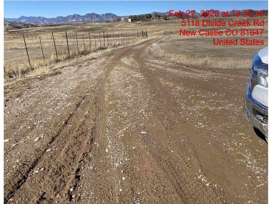
Insufficient Tracking BMPs – Photo #06940
