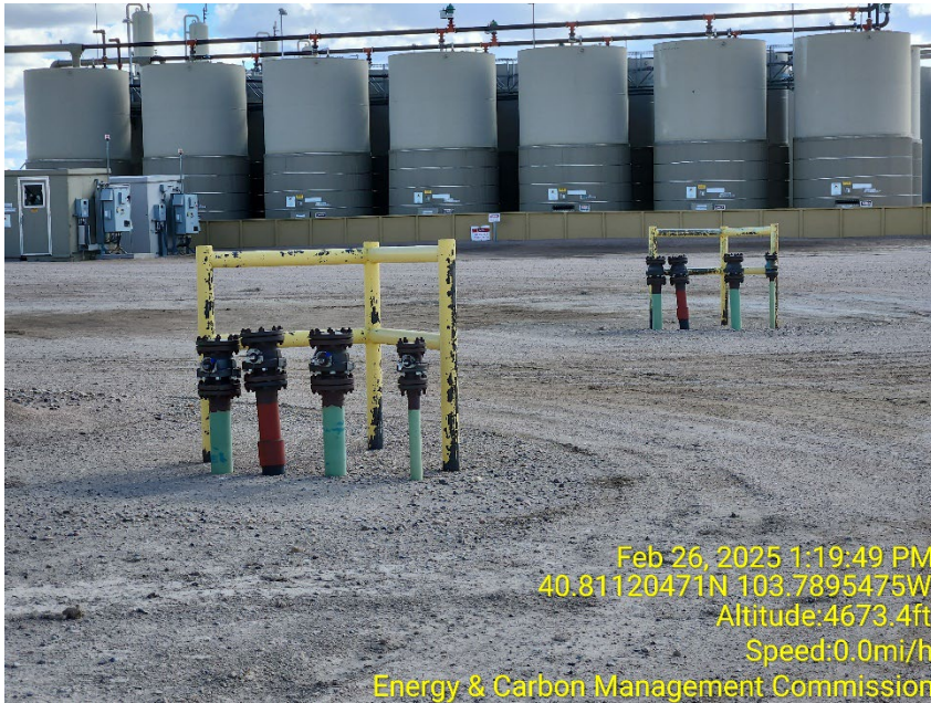
Photo 15 – Unmarked Risers
