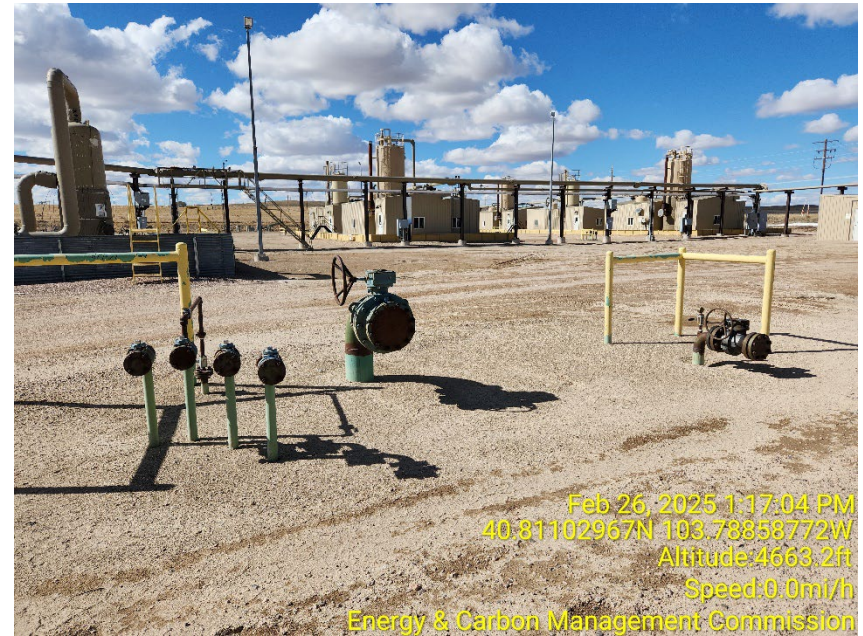
Photo 6 – Unmarked Risers
