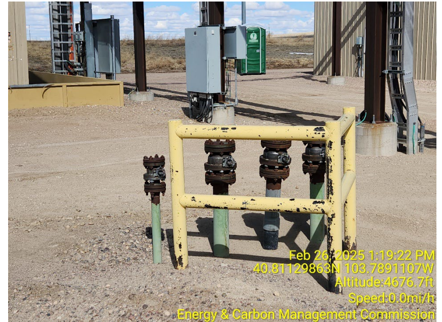
Photo 14 – Unmarked Risers
