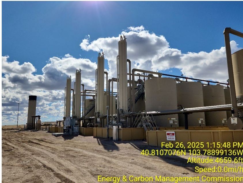
Photo 3 – Tank Battery
