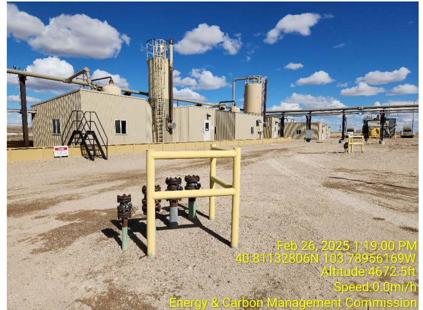
Photo 12 – Unmarked Risers
