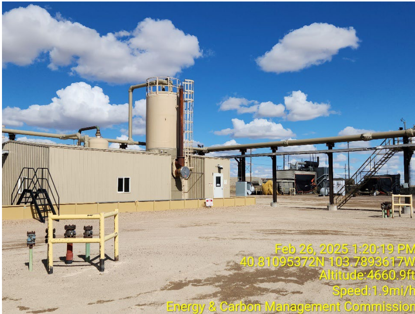
Photo 17 – Unmarked Risers
