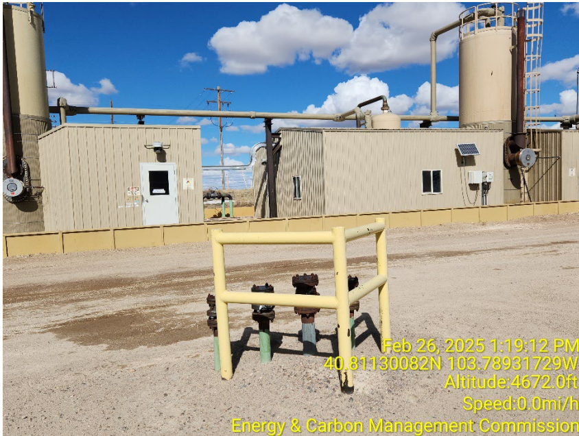
Photo 13 – Unmarked Risers
