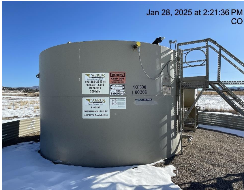
Photo # 1968 From inspection 708905613 conducted on 01/28/2025 Tank is disconnected & not in use/unused equipment
