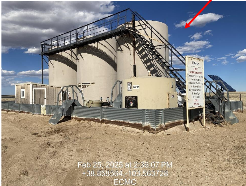
Photo 9 – Tank Battery
