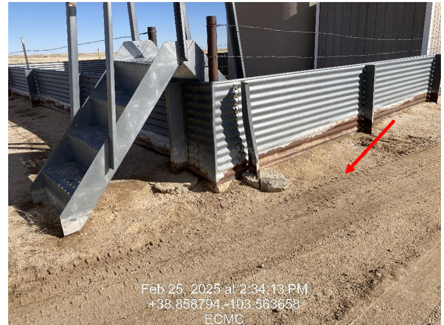
Photo 2 – Area where Spill ID 479428 breached containment
