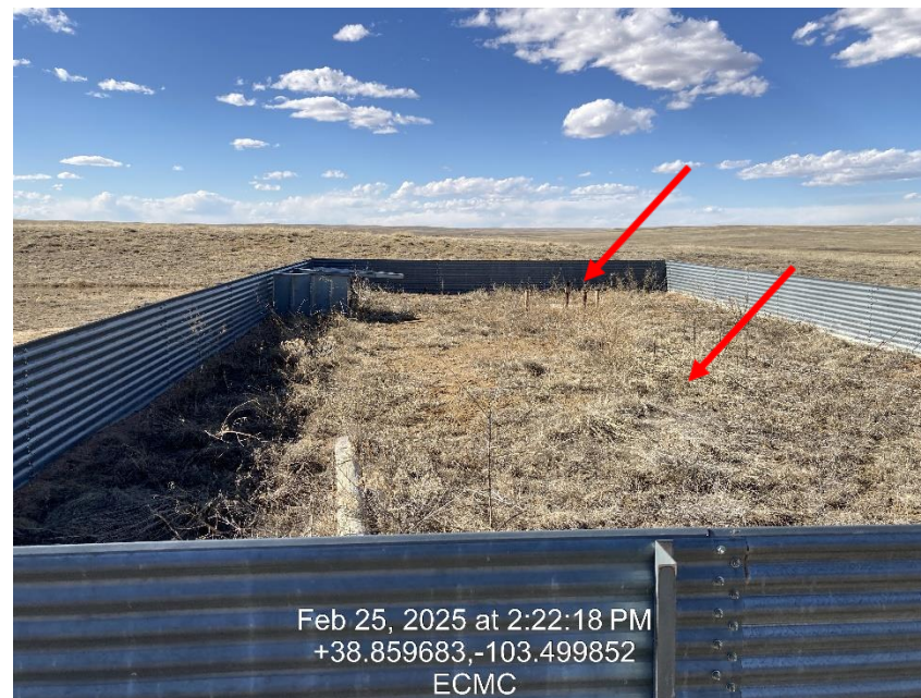
Photo 10 – Unused secondary containment, Unmarked pipes at upper arrow
