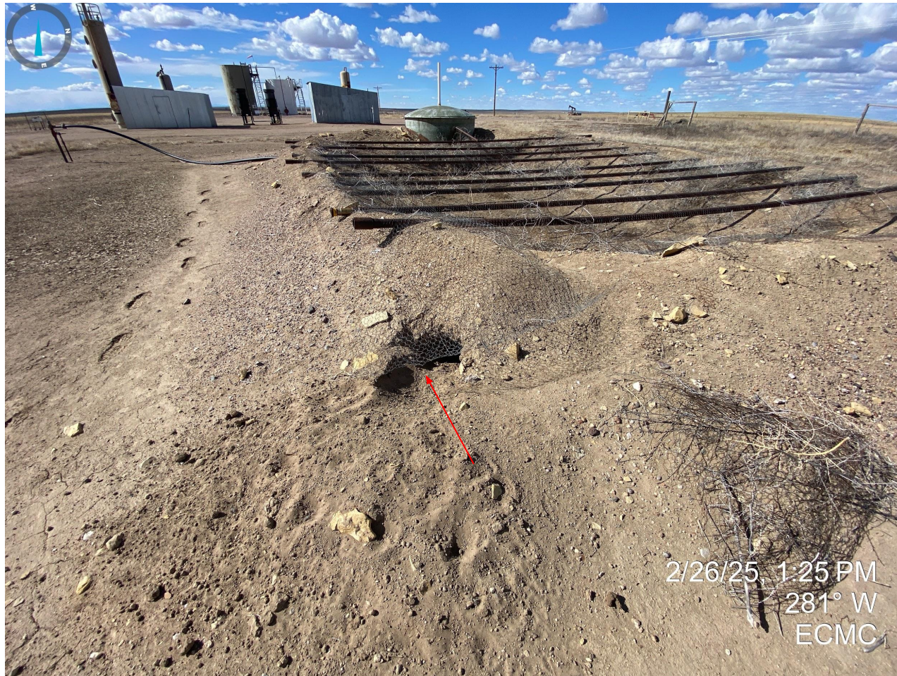
Photo 1. Animal burrow observed at pit berm.
