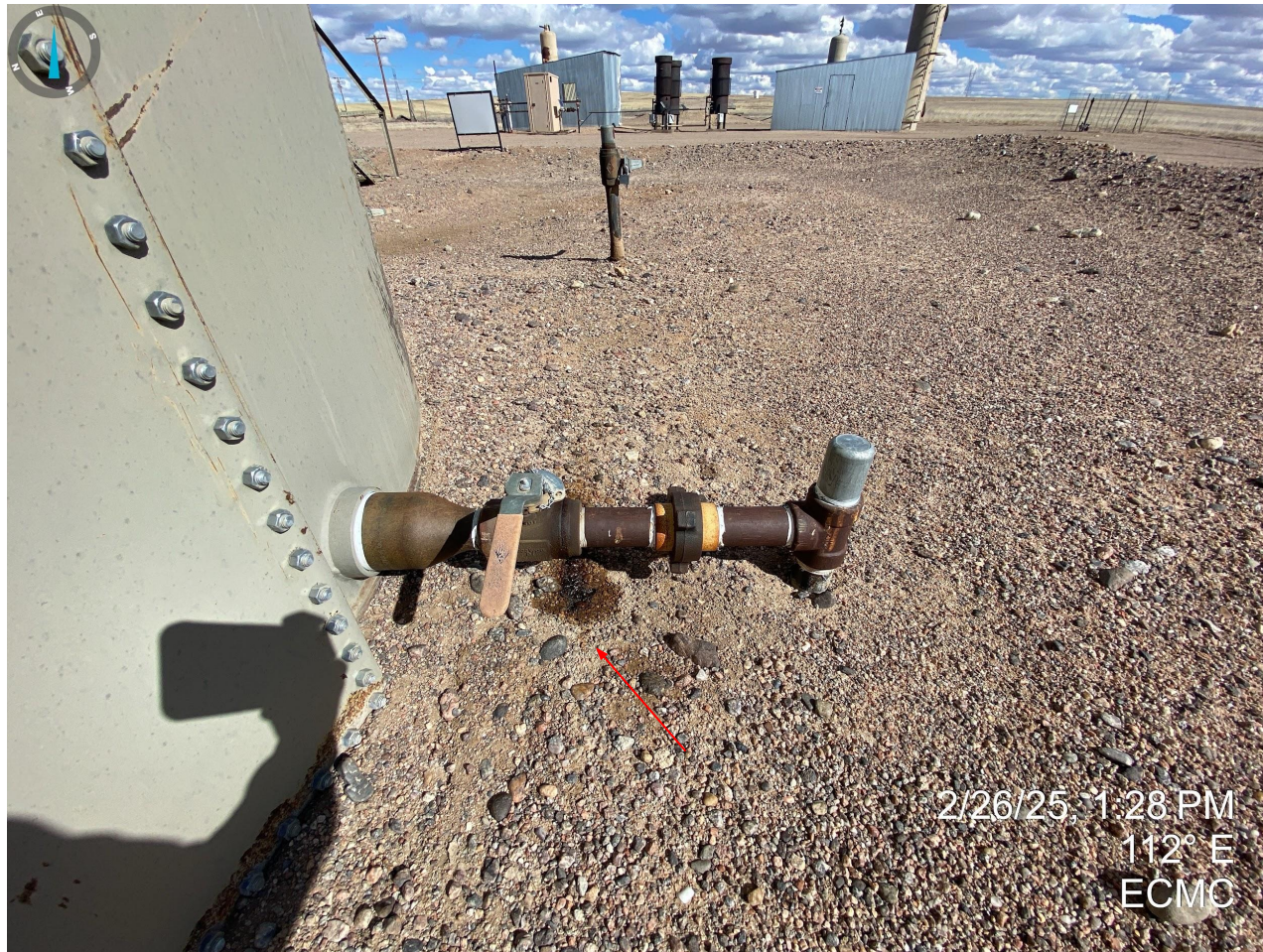
Photo 4. Stained soil and leaky valve at AST.
