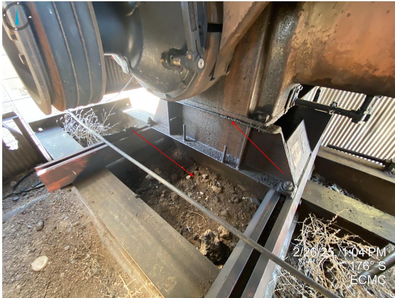
Photo 2. Stained soil and leaking equipment at pumpjack unit.
