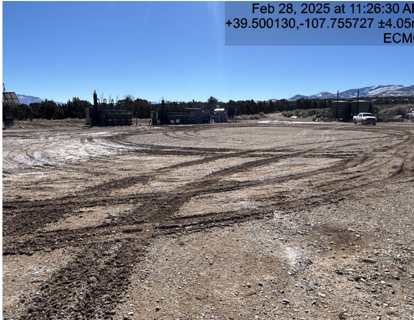
Lack of stabilization/ compaction
