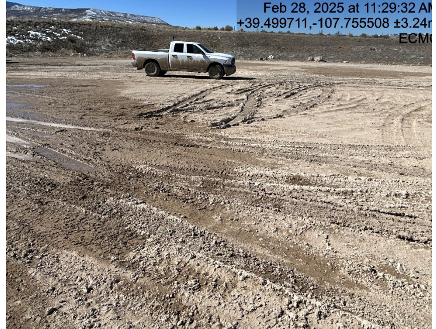
Lack of stabilization/ compaction
