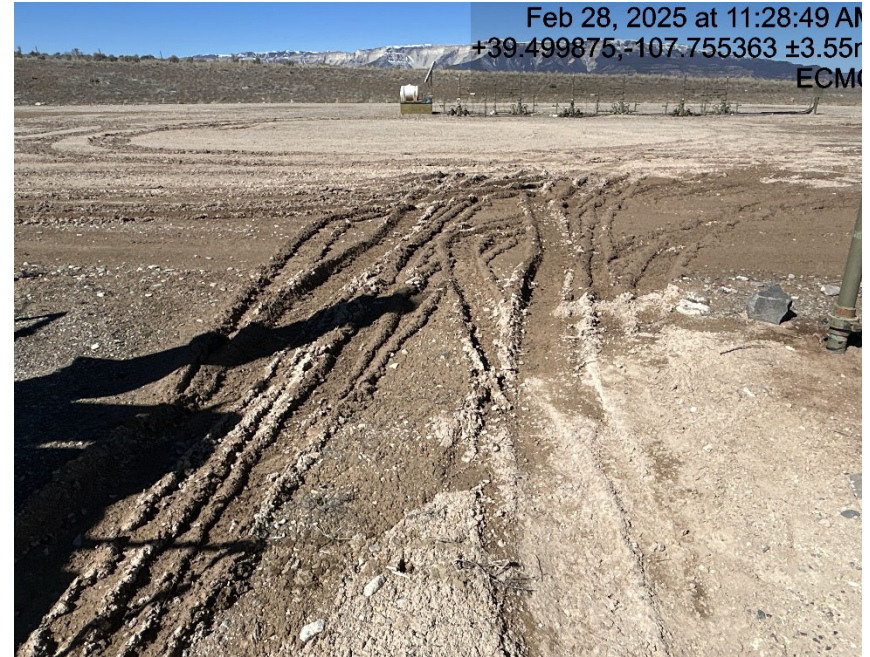
Lack of stabilization/ compaction
