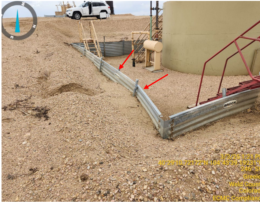
Photo 7: Damage to berm
