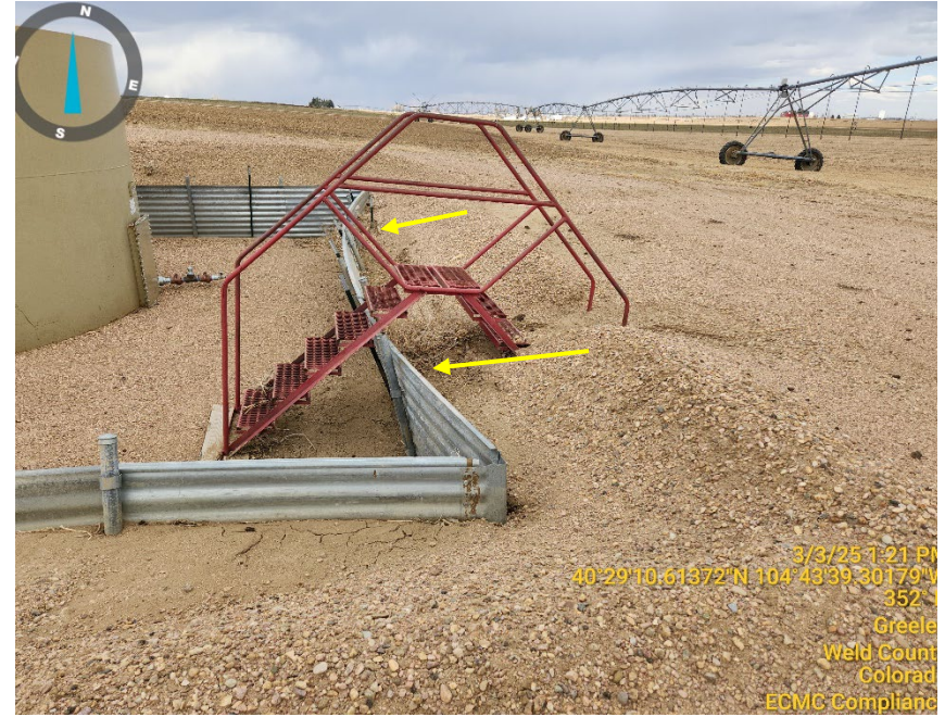
Photo 8: Damage to berm
