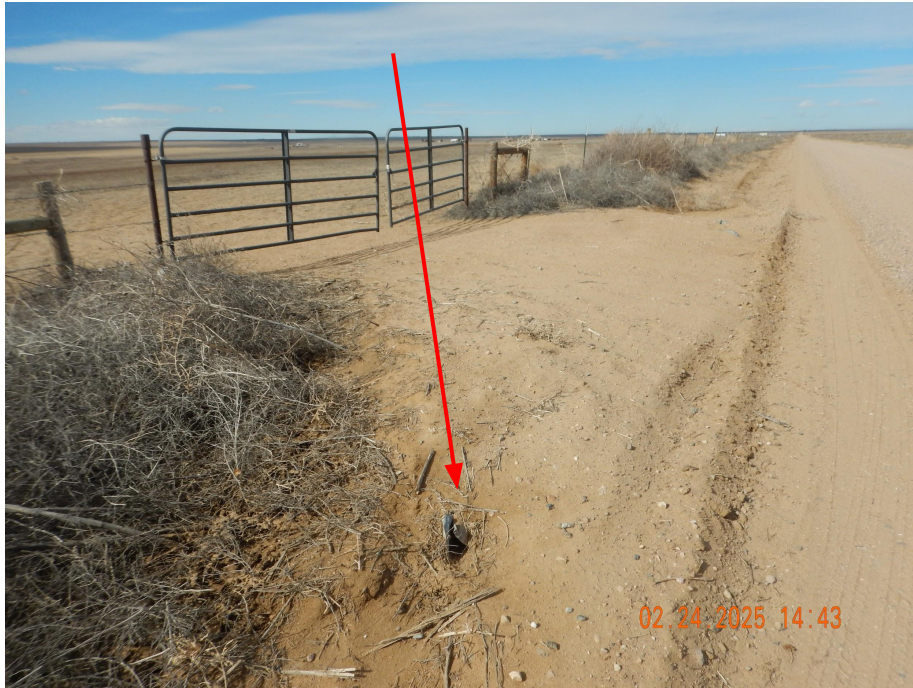
Photo 1. Photo taken from the well location entrance of CR85, facing North. Photo illustrates the culvert has not been removed per Rule 1004.a.
