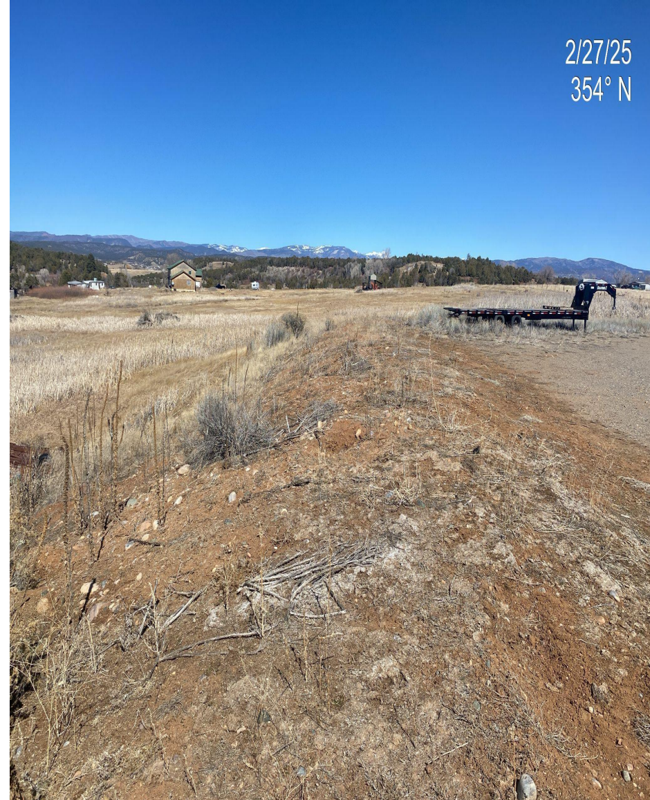
Photo 2. Location cut and fill slopes remain with mostly bare soils and minimal desirable veg. Hydro mulch has worn off and seeding efforts do not appear successful, no new desirable vegetation growth observed. Weeds appear to be treated/managed at this time.
