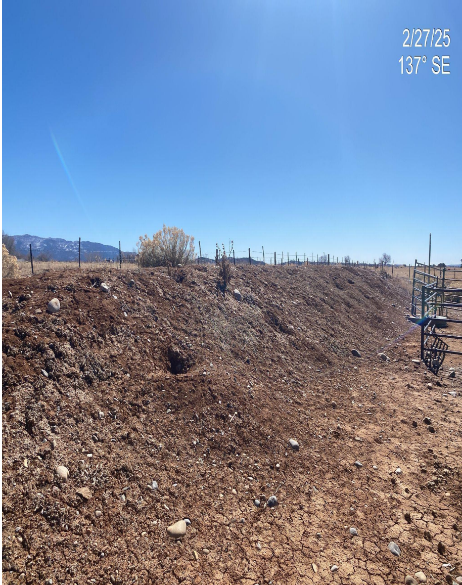
Photo 2. Location cut and fill slopes remain with mostly bare soils and minimal desirable veg. Hydro mulch has worn off and seeding efforts do not appear successful, no new desirable vegetation growth observed. Weeds appear to be treated/managed at this time.
