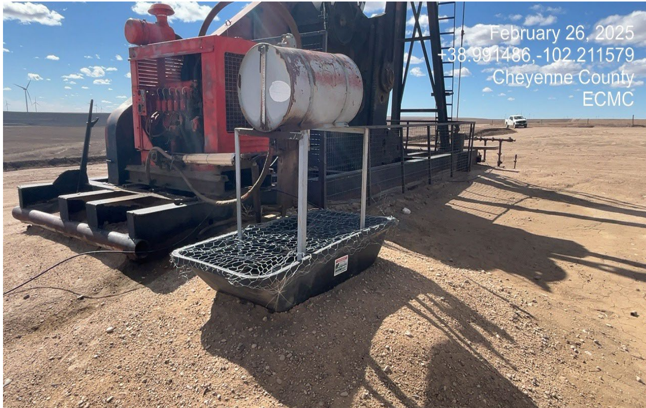
Photo 5. The containment has woven wire for wildlife protections.
