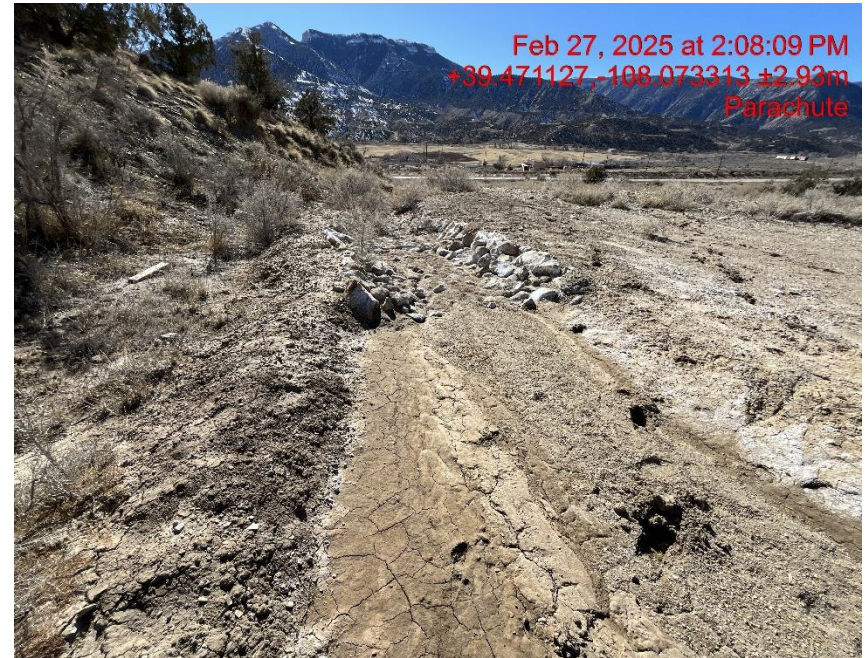
Photo # 6118 Ditch/Rip Rap needs maintenance
