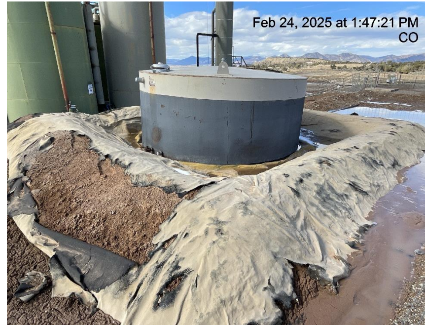
Photo # 8430 Secondary containment inadequate/does not comply with CECMC rules
