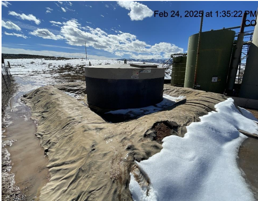
Photo # 8429 Secondary containment inadequate/does not comply with CECMC rules
