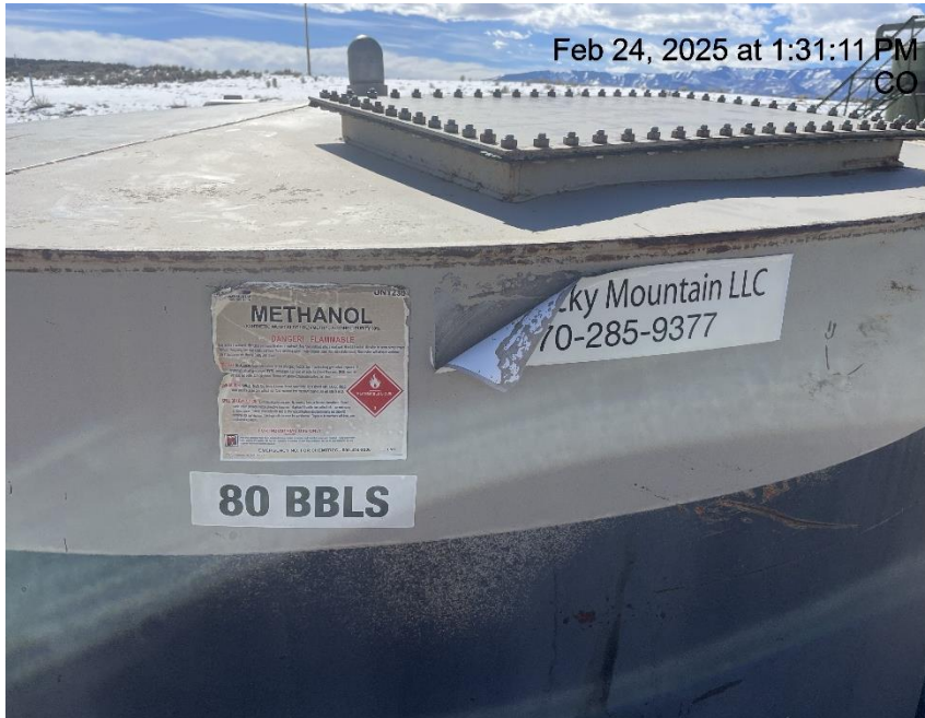
Photo # 8419 Tank label damaged/some required information is becoming illegible & tank capacity incorrect /not in compliance with CECMC rules
