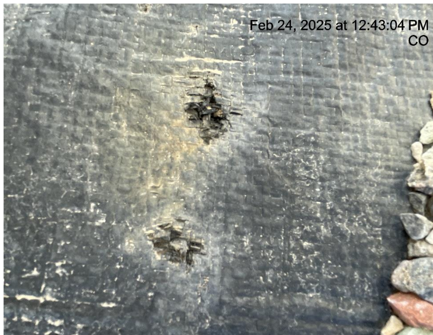
Photo # 8232 Holes in liner/liner needs maintenance
