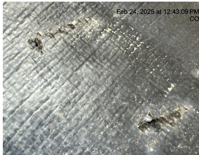
Photo # 8233 Holes in liner/liner needs maintenance
