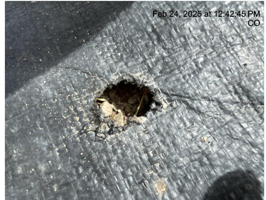
Photo # 8231 Hole in liner/liner needs maintenance
