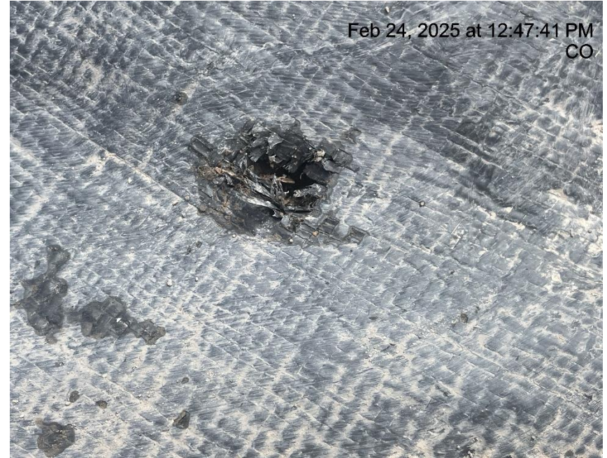
Photo # 8235 Hole in liner/liner needs maintenance
