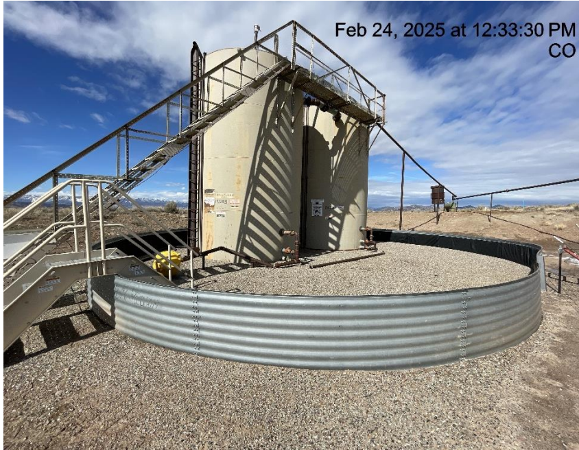
Photo # 8236 Battery lacks required signage
