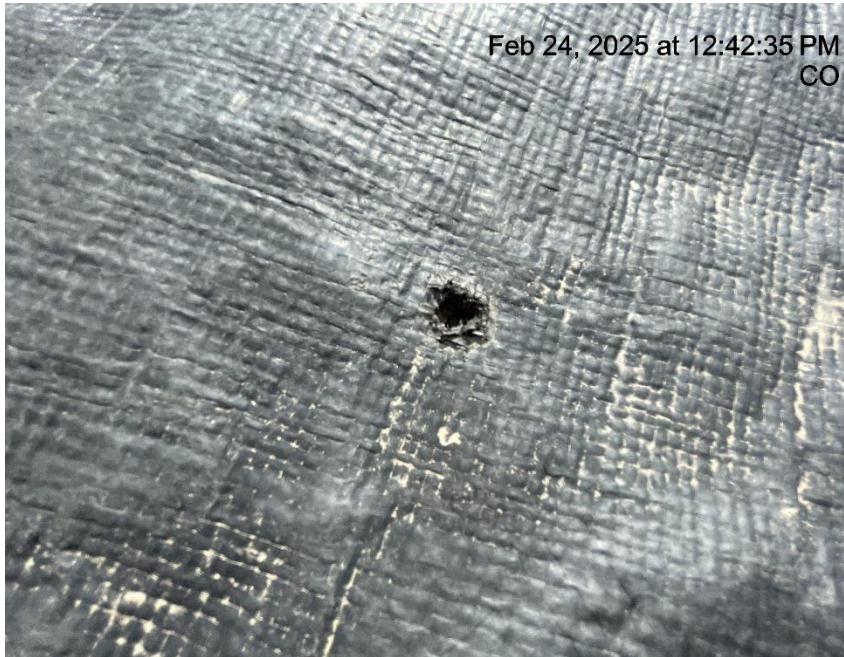
Photo # 8230 Hole in liner/liner needs maintenance
