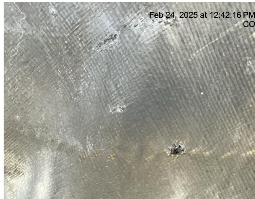
Photo # 8229 Hole in liner/liner needs maintenance
