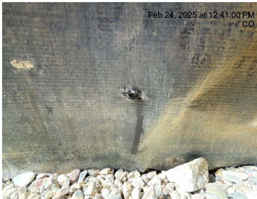
Photo # 8228 Hole in liner/liner needs maintenance
