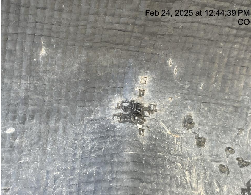
Photo # 8234 Hole in liner/liner needs maintenance
