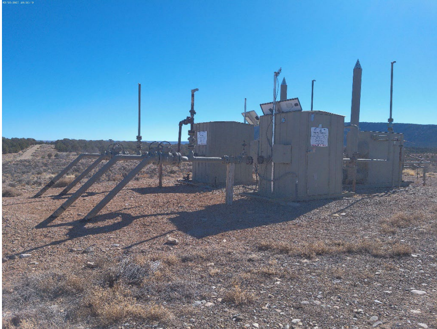
Separators and Meter housings
