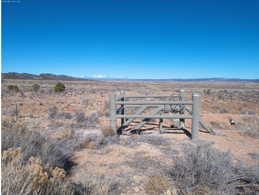
Off location Flowline Riser and Valve
