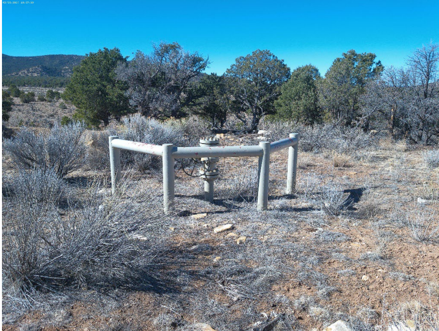
Off location Flowline Riser and Valve
