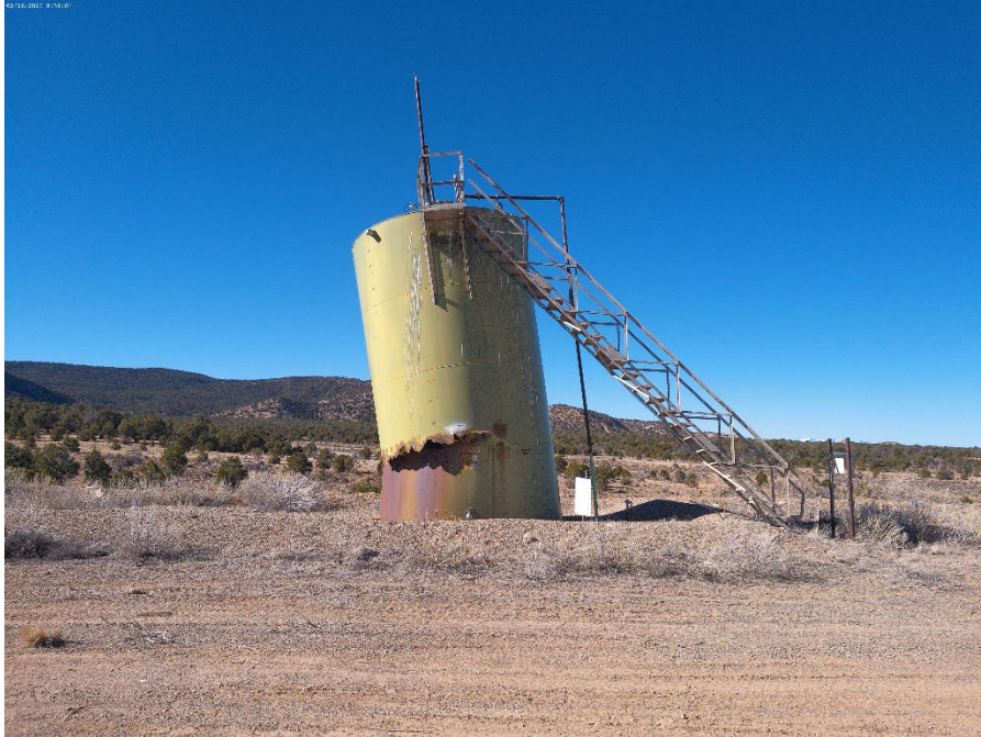
Tank battery rusted and collapsed.
