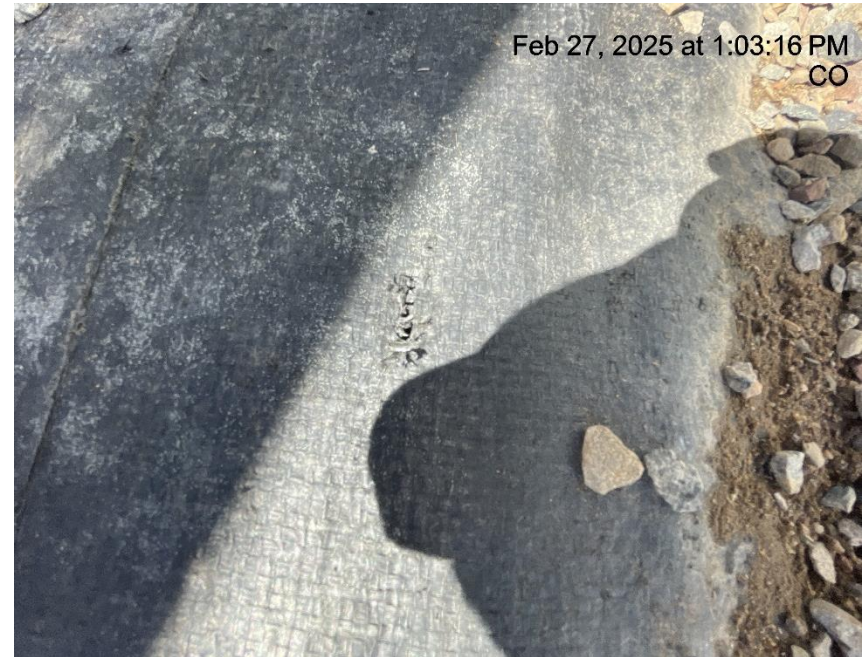
Photo # 155 Hole in liner/liner needs maintenance
