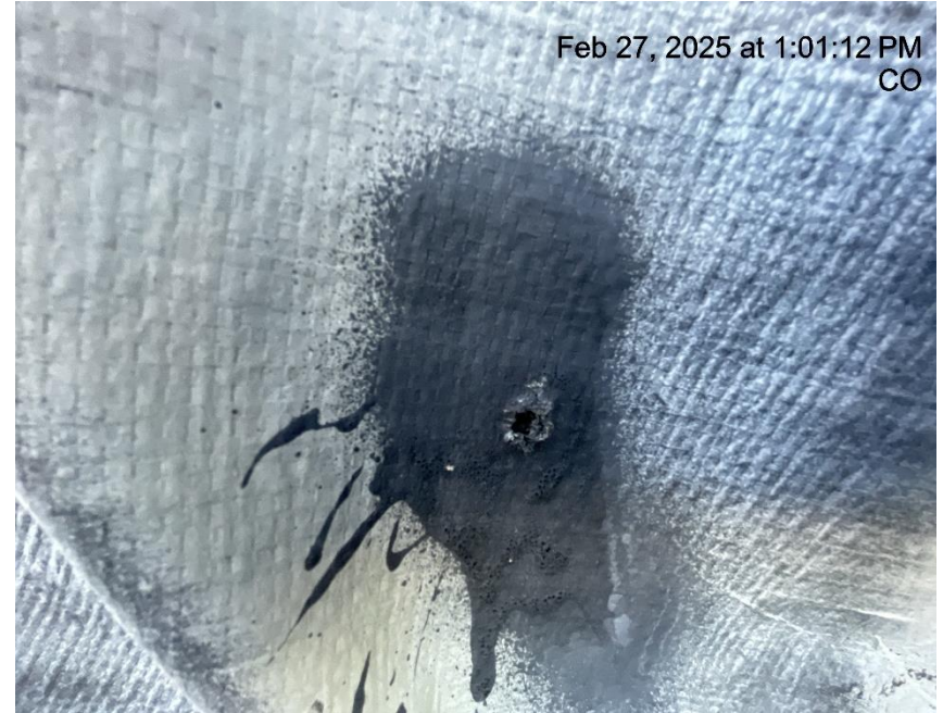
Photo # 157 Hole in liner/liner needs maintenance
