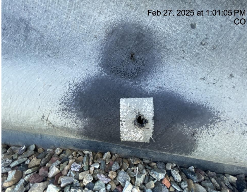
Photo # 156 Holes in liner/liner needs maintenance
