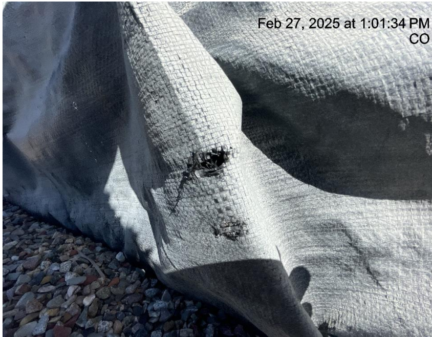
Photo # 158 Holes in liner/liner needs maintenance
