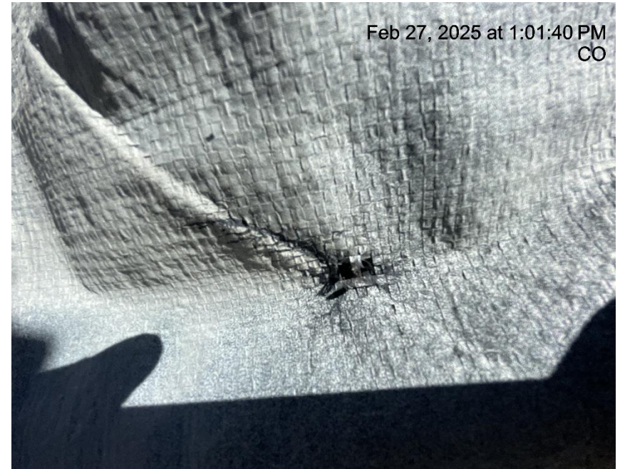
Photo # 159 Hole in liner/liner needs maintenance
